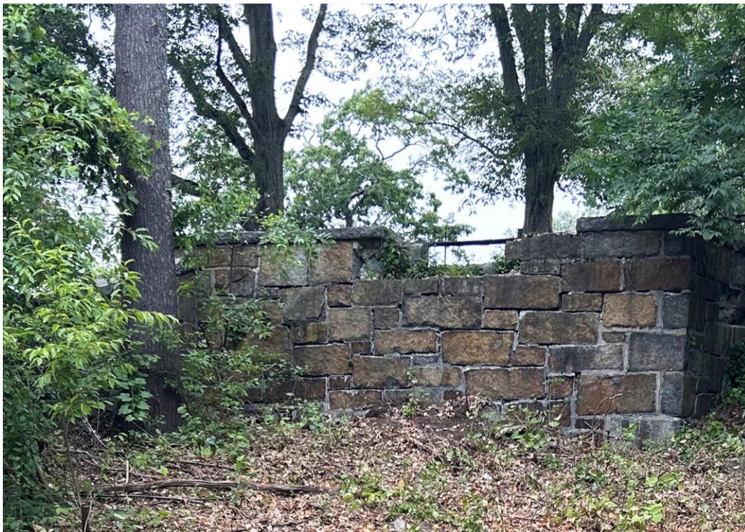
The walls on either side of the stairs have been power washed, repaired and repointed. The photo above shows the completed work and the photo below shows the before condition.
