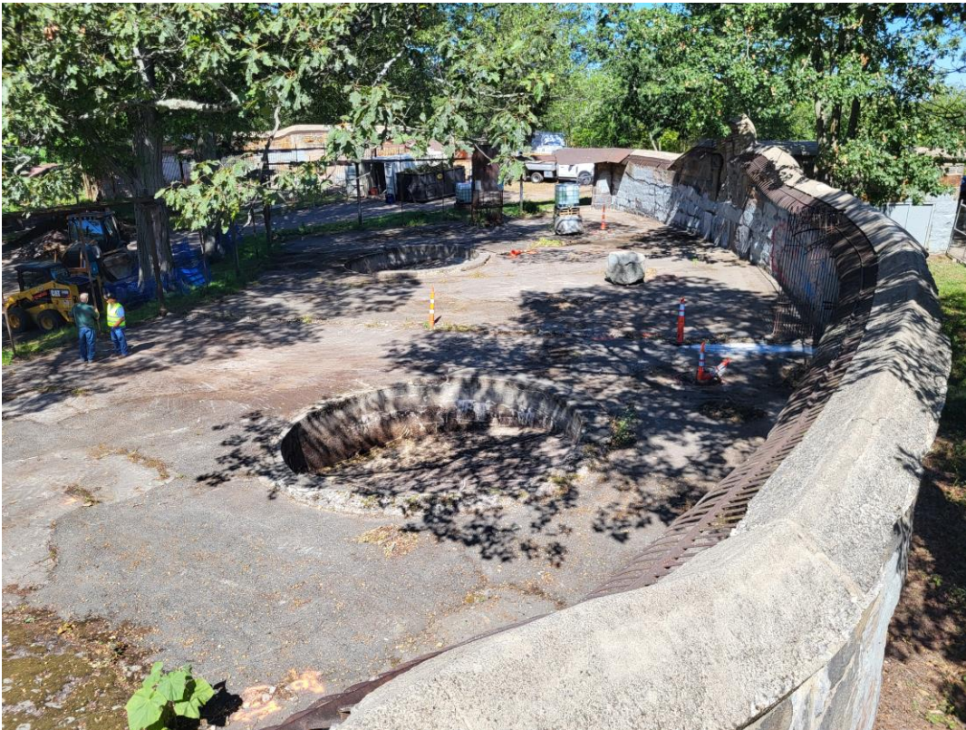
The cap at the top of the wall has been power washed in preparation for filling in cracks
