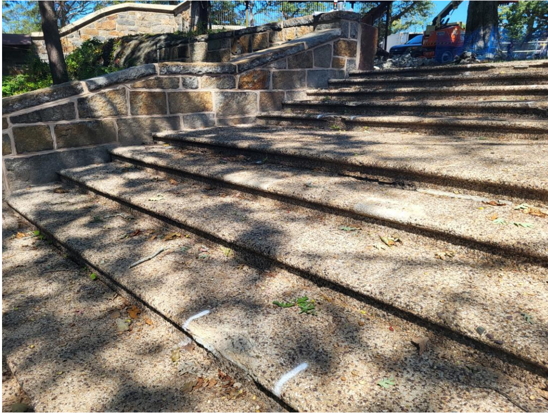
The stairs have been power washed in preparation for filling gaps and cracks
