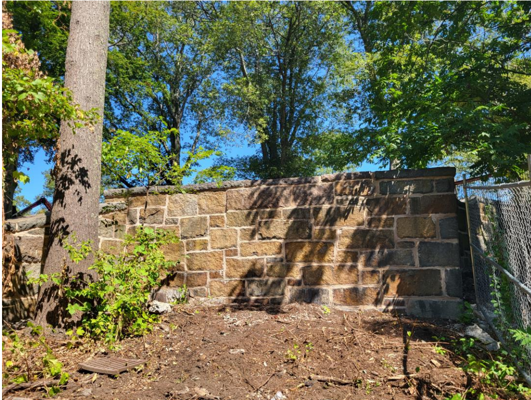
The walls on either side of the stairs have been power washed, repaired and repointed. The photo above shows the completed work and the photo below shows the before condition.
