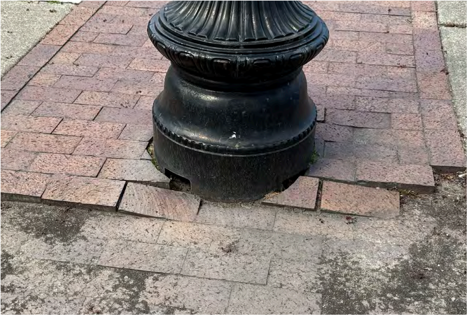
2 Cracking brick pavings; rat holes at the base of the pole lights.
