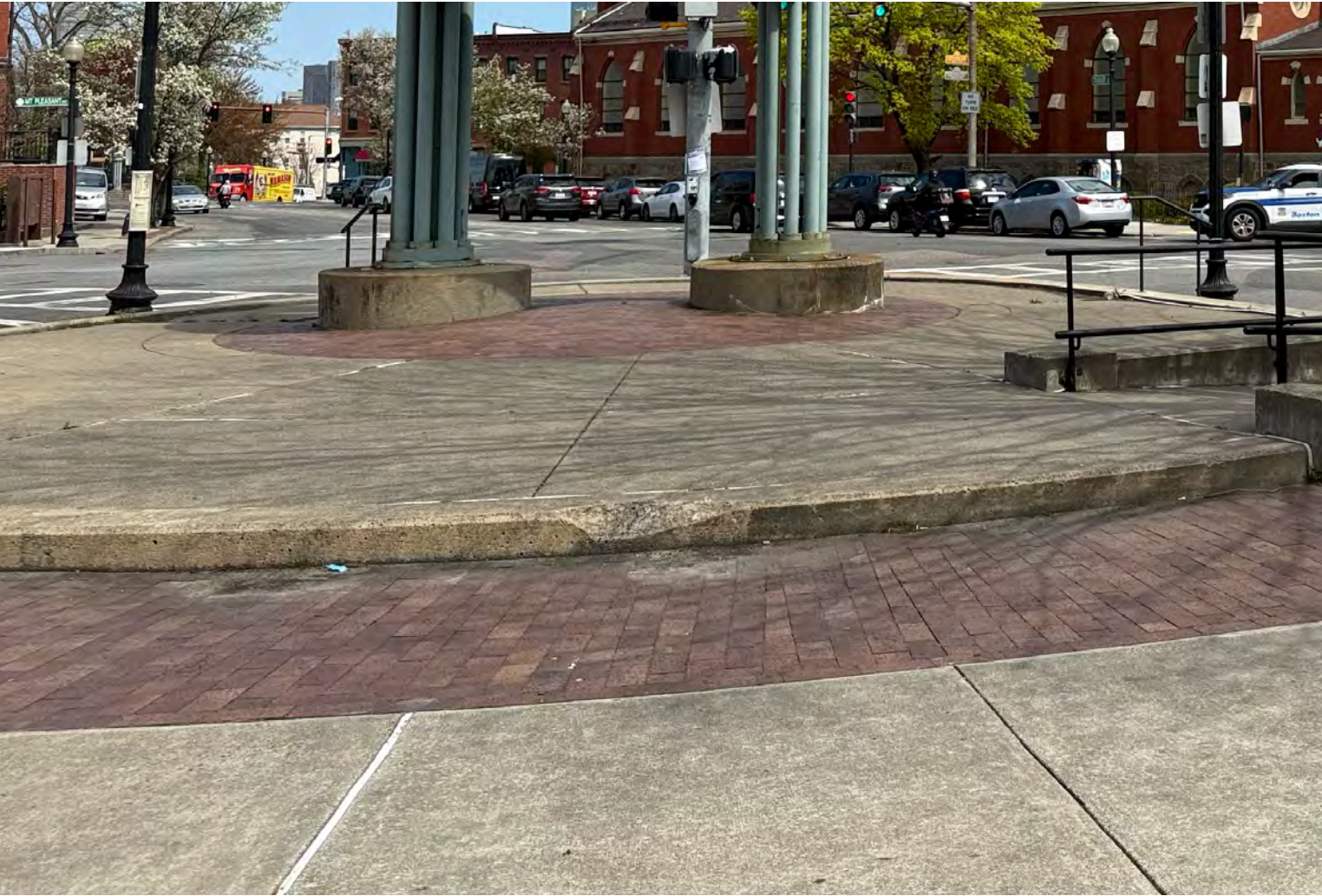
1 Multiple steps within plaza creating potential trip hazard. Ramps project into plaza further restricting and obstructing space.
