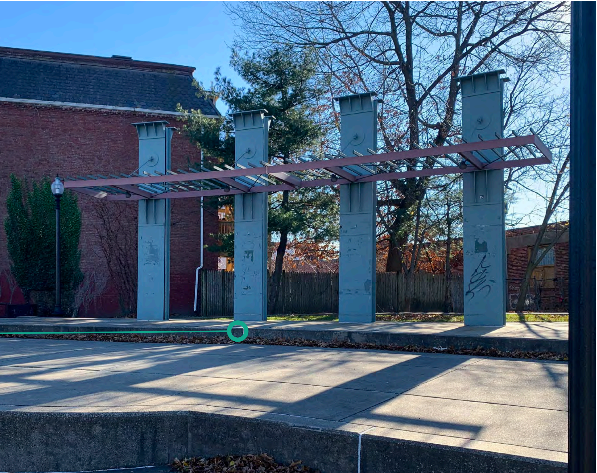
1 Fading paint at stage back-drop, non-functioning lights, paving cracks.
