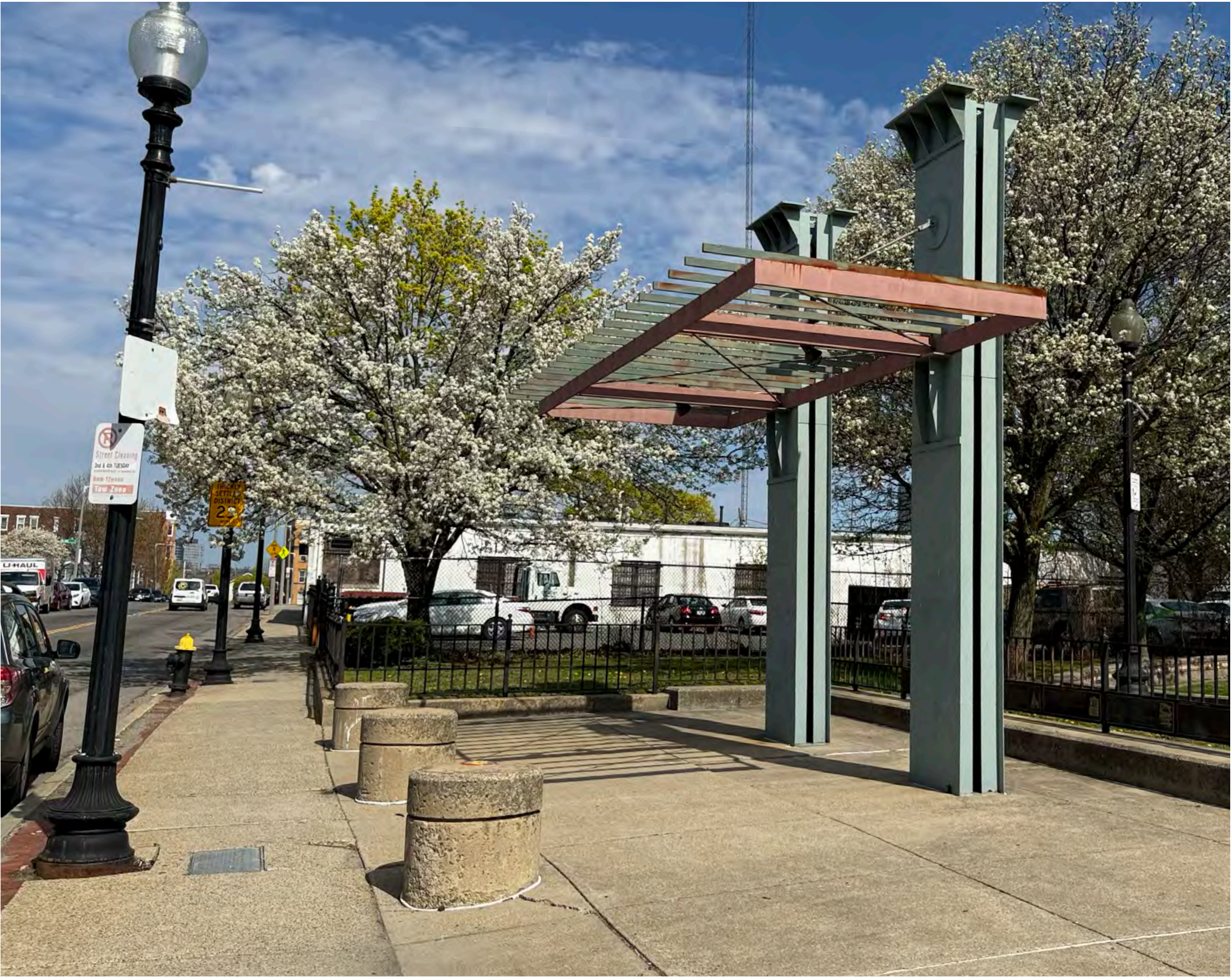
1 Bollards & shade structure do not contribute to bus stop and restrict site lines in park. Cracking and heaving of concrete paving. No defined seating.
