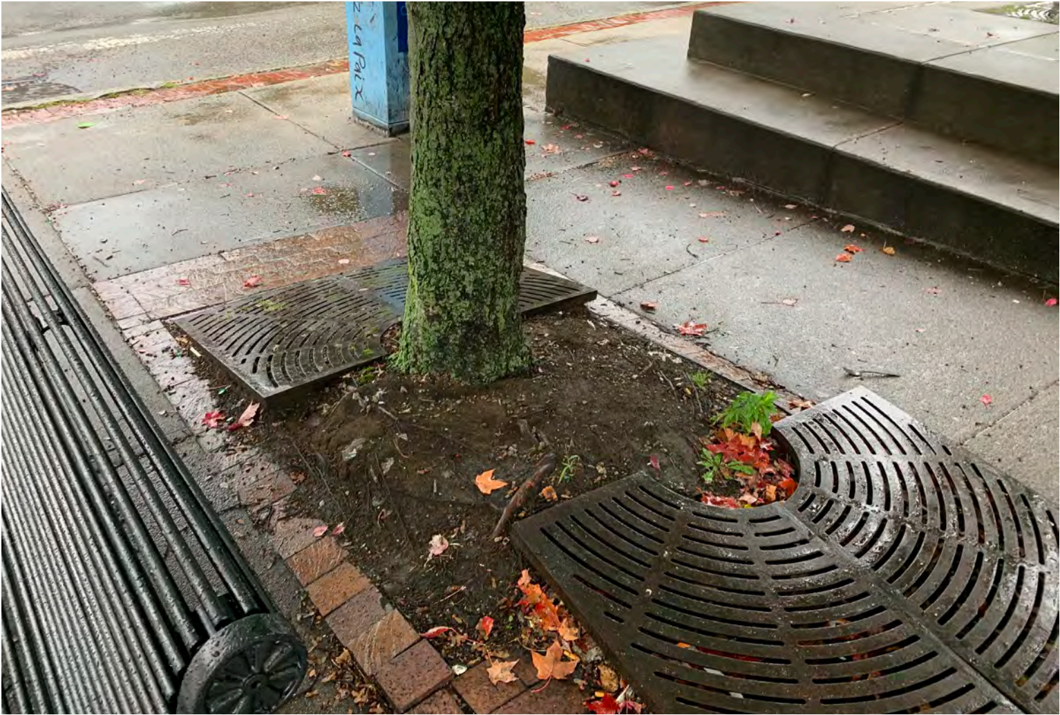
2 Tree grate not adjusted for tree growth. Tree is root-bound and heaving paving and grate.
