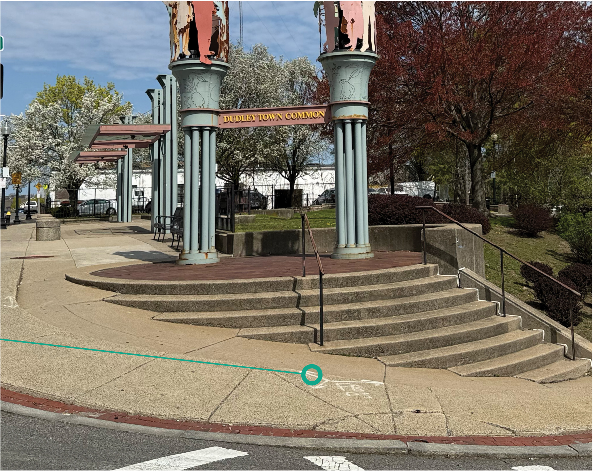
1 Uneven concrete paving has compromised the ADA ramp’s functionality and poses a potential trip hazard.
