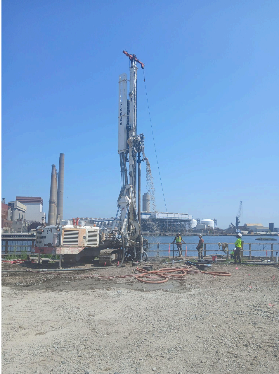
Micropile installation in progress.
