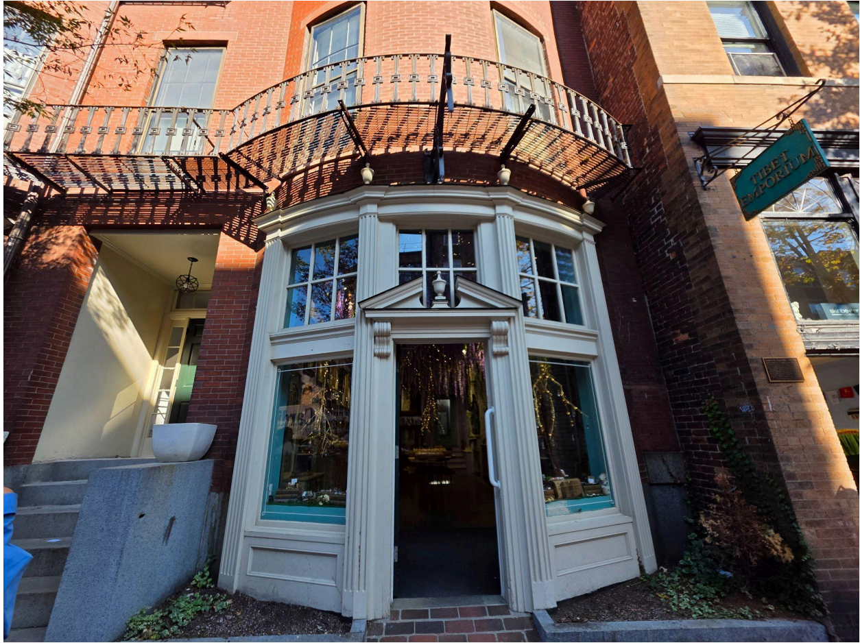
Existing Conditions of 105 Charles St Boston, MA 02114
