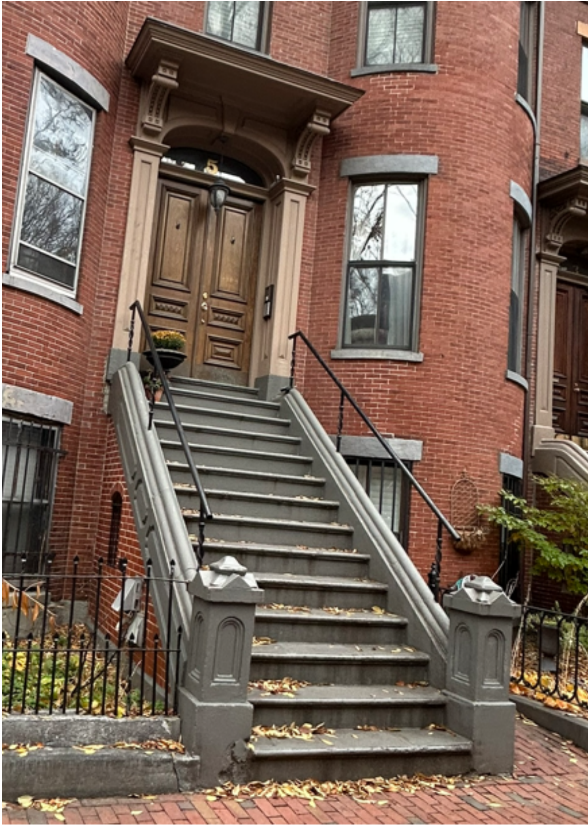
Entry Stair & Parlor Door Inspiration (3-5 Wellington)
