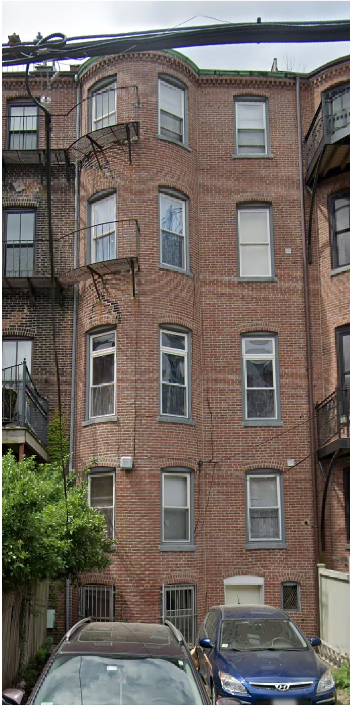
Rear Alley Facade
