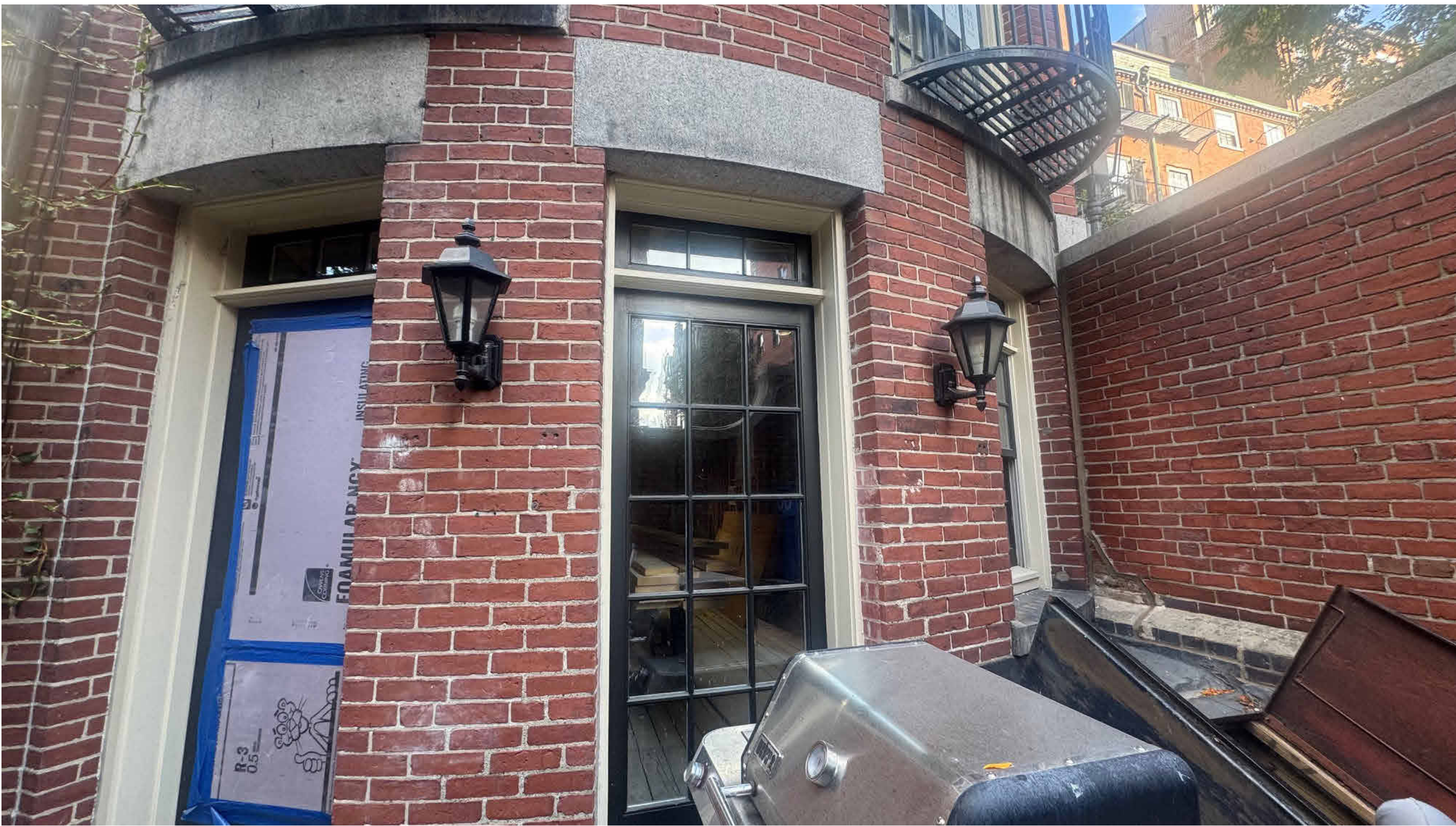
EXISTING NON-HISTORIC WINDOW/DOORS WITH TRANSOMS FROM INSIDE GARDEN
