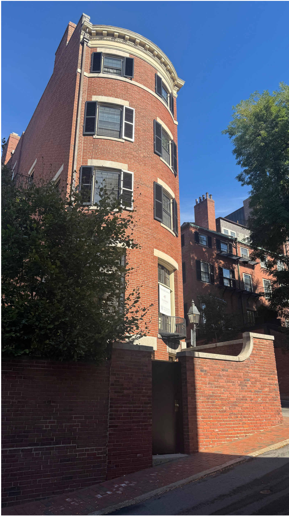
VIEW 2 (FROM BRANCH STREET)
