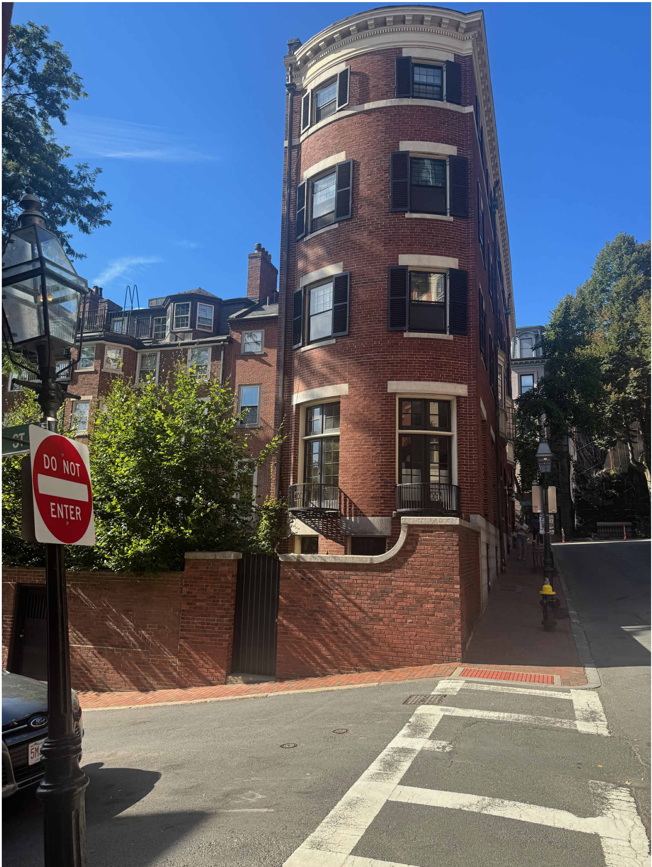
VIEW FROM BRANCH STREET & SPRUCE STREET JUNCTION
