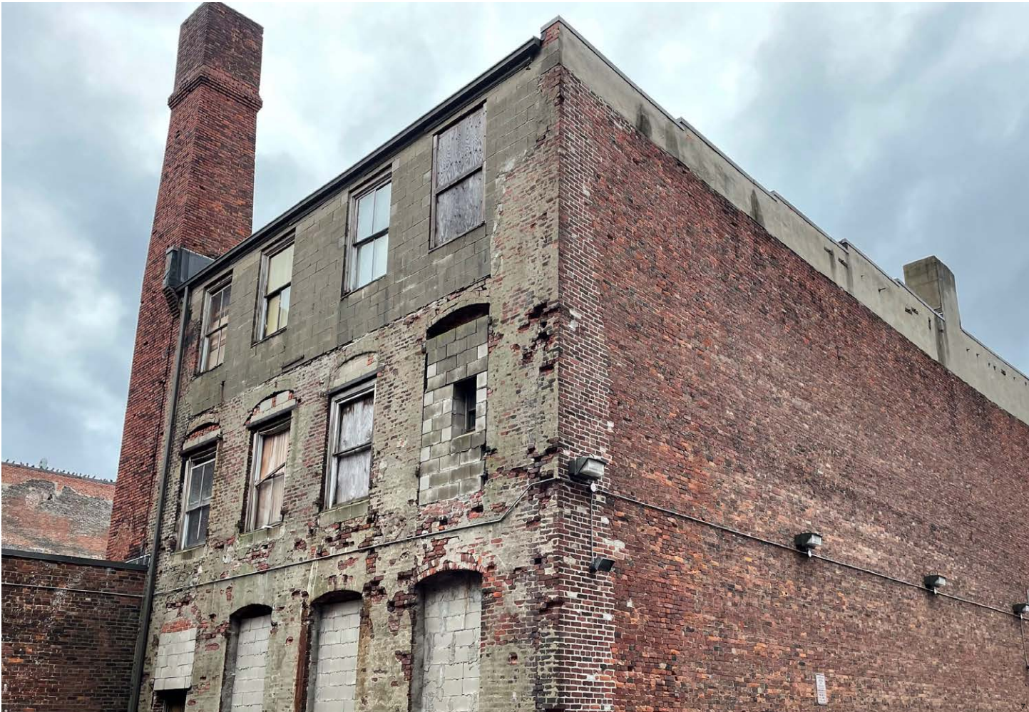
Figure Y: Rear facade of 52 Plympton Street. The rear facade exhibits significant structural issues consistent with the building's overall state of decline. This includes widespread masonry deterioration and evidence of structural settlement. These conditions, which will be further detailed in a forthcoming structural engineering report, contribute to the building's compromised integrity and the infeasibility of its restoration.
