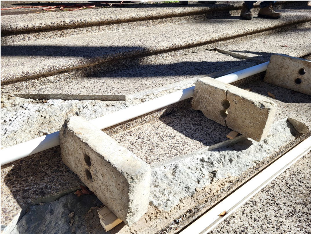
Concrete formwork in place for the stair repairs
