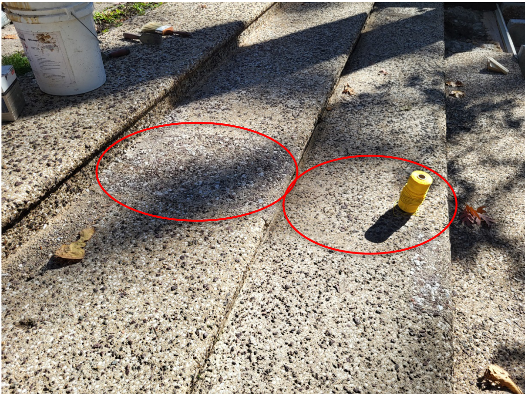
Sample areas where the new concrete has been poured for the stair repair
