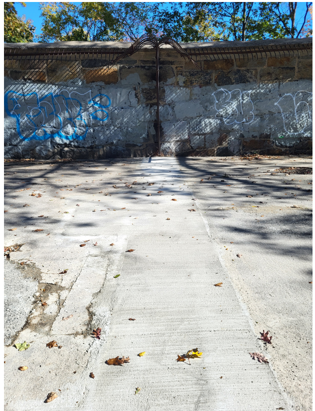
Concrete repairs ongoing between Cages 2 and 3 (prepping for new concrete – left – and the new concrete – right)
