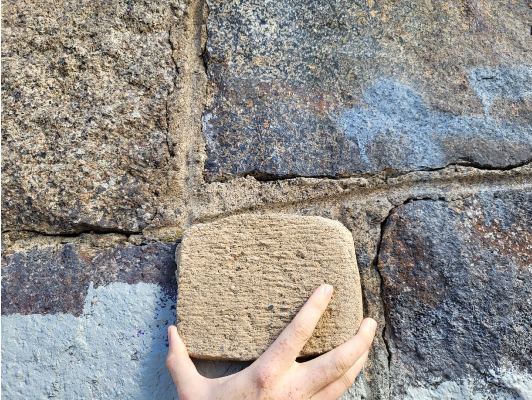
The contractor developed a custom mortar mix to match the existing mortar as closely as possible
