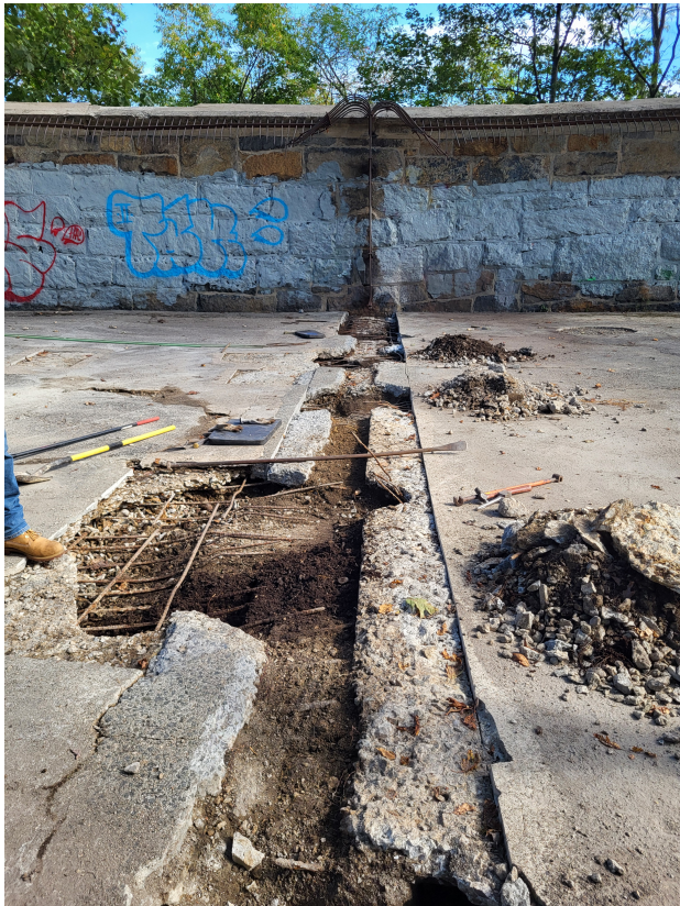
Concrete repairs ongoing between Cages 2 and 3 (prepping for new concrete – left – and the new concrete – right)
