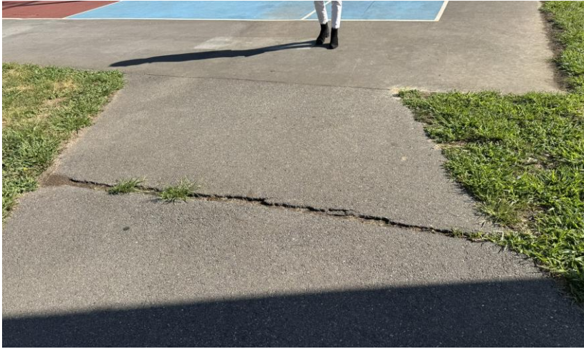
CRACKS IN PAVEMENT
