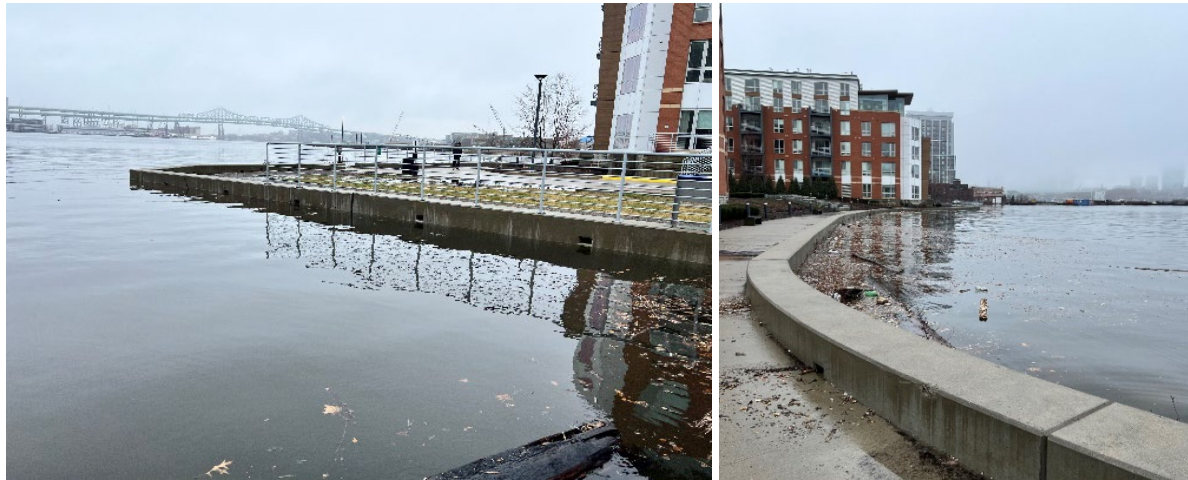
Figure 3. Flood waters reaching the scuppers on the seawall at the Boston East Apartments at 126 Border Street during January 2024. Coupled with a king tide event, or a few more inches of rain and the seawall's elevation would not have blocked the flood waters. Weston & Sampson, 2024.
