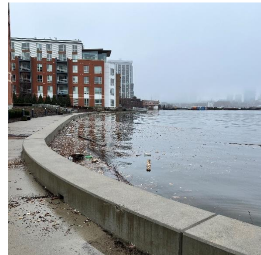
Figure 23. Flood waters reaching the scuppers on the seawall at the Boston East Apartments at 126 Border Street during January 2024. Coupled with a king tide event, or a few more inches of rain and the seawall's elevation would not have blocked the flood waters. Weston & Sampson, 2024.
