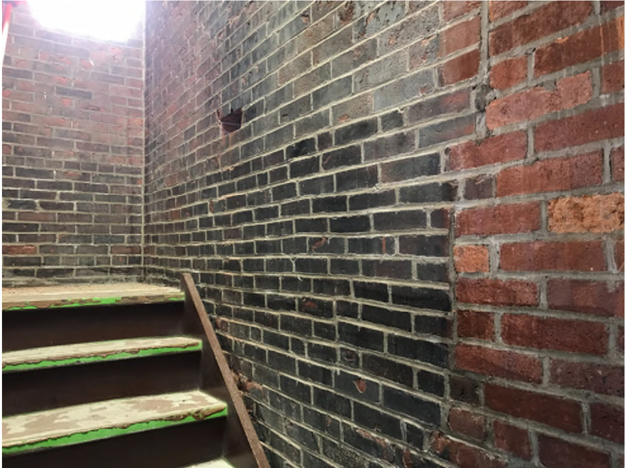
Photograph #9 – This photograph shows a common example of the condition of brick at the Eastern wall at the inside of the Northeast stair. The brick is intact with full joints that appear to have been previously repointed. Additionally, a different color and texture of brick occur at the righthand side of the photo which appear to be an infill or a previously existing door. This may be indication that this wall was a common “party” wall with a taller existing structure located at 401 Shawmut Avenue that has since been demolished. Also in this photograph is the location where brick was sampled for testing.
