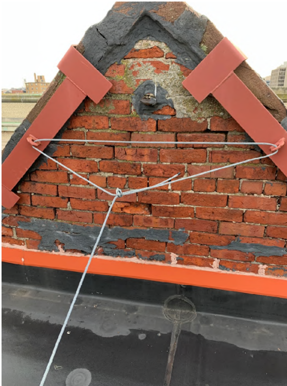
Photograph #1 – This photo shows a typical existing masonry parapet condition with existing masonry in disintegrated state along with external bracing required due to the deterioration.
