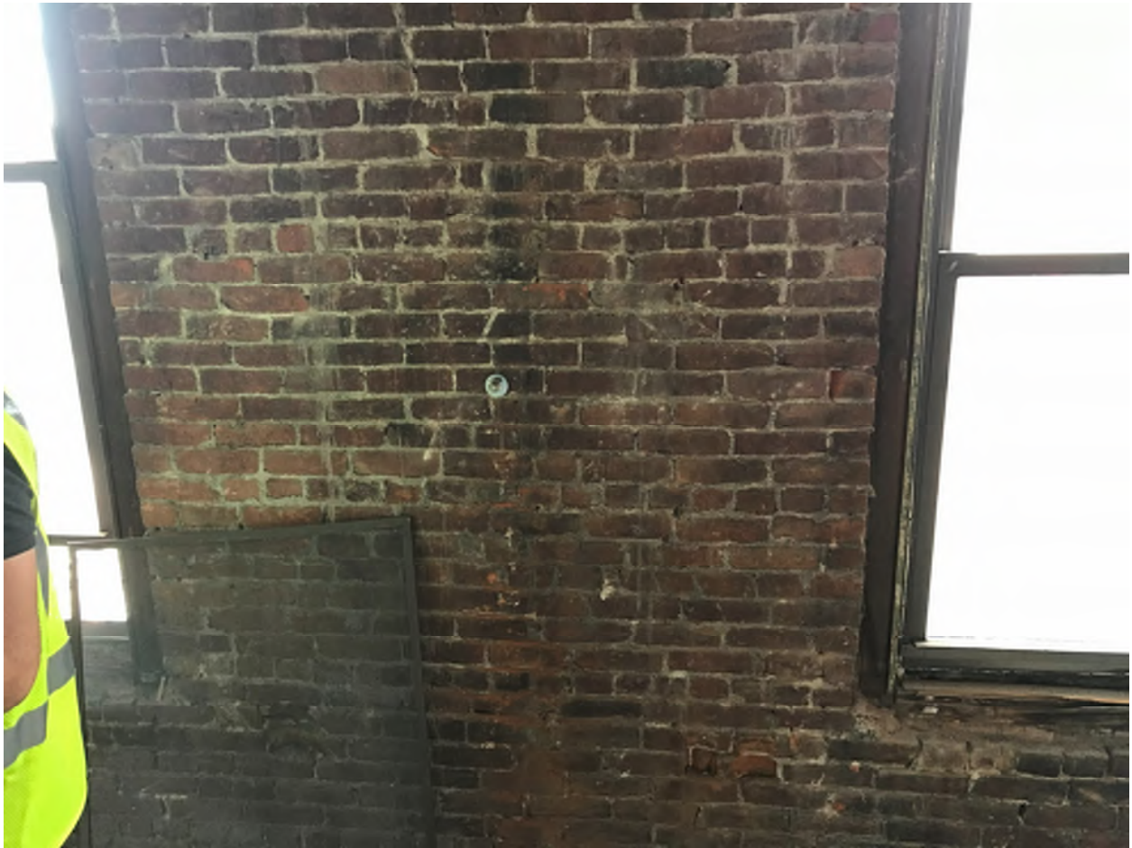
Photograph #8 - This photograph shows another masonry pier between windows on the Southern Shawmut Avenue elevation at the fifth-floor level. The brick pier here remains with intact brick and mortar, and it is noted that header courses occur within the brick pier as well. The construction at the base of the pier / at windowsill level is in good condition without open joints and significant mortar recession.
