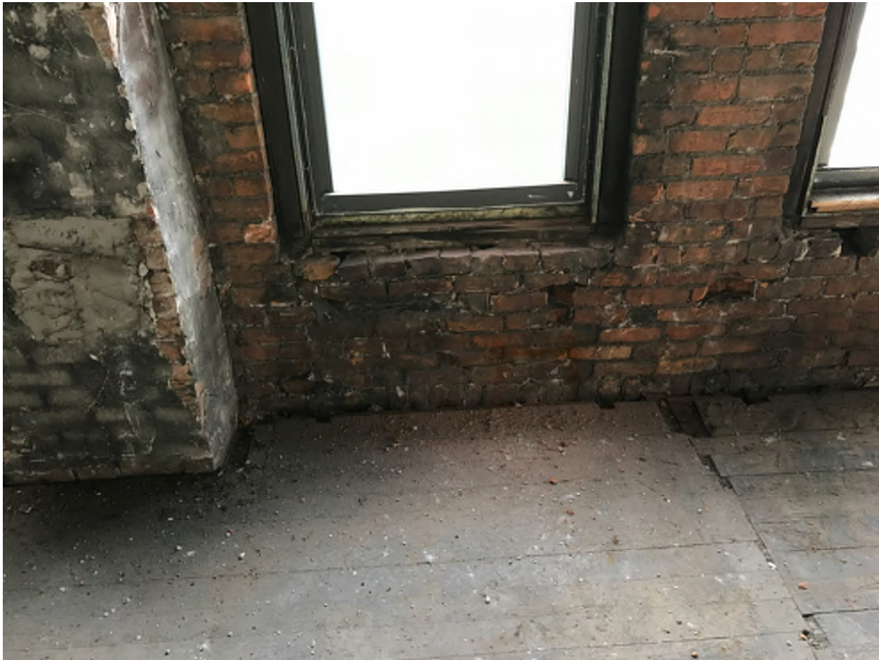
Photograph #10 -This photograph shows the masonry below windowsill at the Southern Shawmut Avenue side of the building on the third-floor level. Some of the locations of masonry below windowsill in the lower portions of the building exhibit mortar recession and some loose brick. However, this sill is still in a relatively better condition than that which is shown in Photograph #3 above. This sill has more mortar in joints with some dusting and only a few open joints. All masonry within 8" of the jambs and sills of window openings I recommended to be repointed, and a few locations will require some brick and mortar rebuilding.
