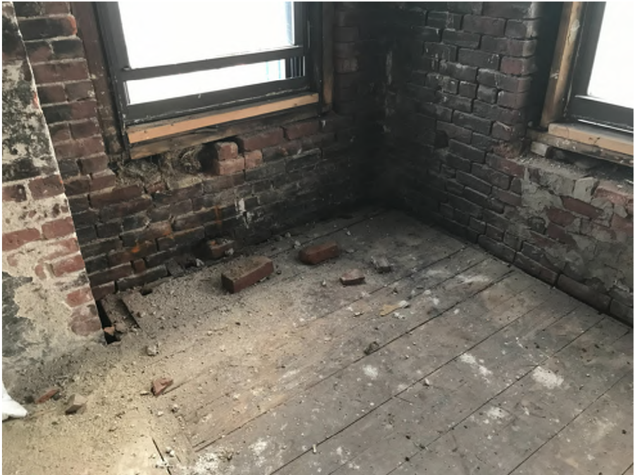
Photograph #3 – This photograph shows the masonry below windowsill at the Southwest corner of the building on the sixth-floor level. Both the sill on the lefthand side and the field of wall around the corner on the righthand side have excessive mortar recession and the righthand sill has loose and missing brick.
