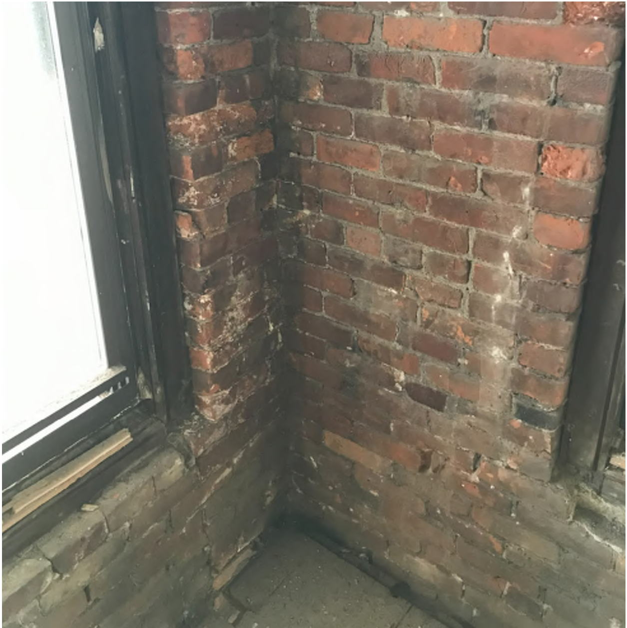
Photograph #6 – This photograph shows the inside face at the Southeast corner of the building on the fifth floor, similar to Photograph #3 which was taken at the sixth floor. This section of wall is in comparatively better condition with intact brick and mortar joints without much disintegration / dusting or mortar. The area under the windowsills is intact with a few open head joints.
