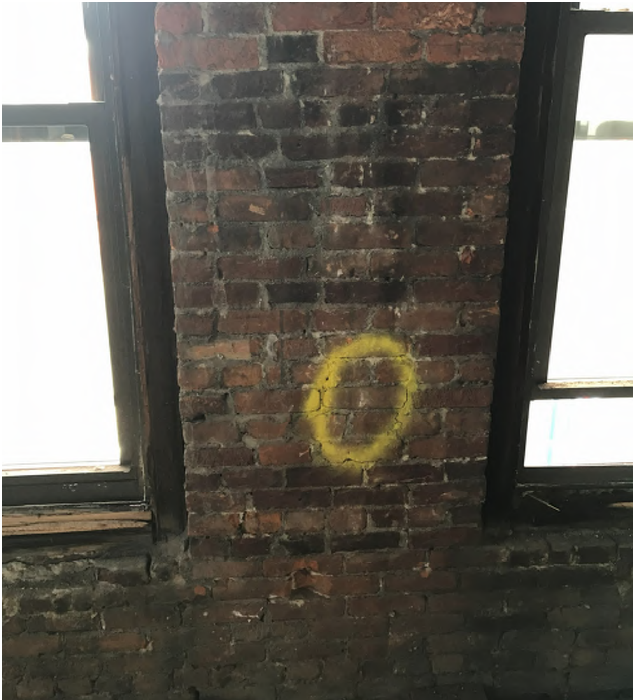
Photograph #7 – This photograph shows a masonry pier between windows on the Southern Shawmut Avenue elevation at the fifth-floor level. The brick pier appears with intact brick and mortar, and it is noted that header courses occur within the brick pier as well. Some open joints occur near the base of the pier / at windowsill level.
