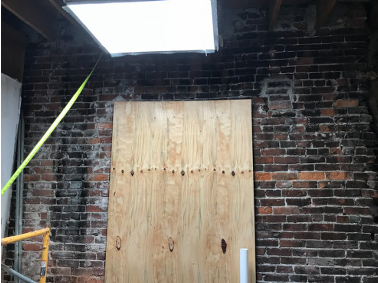
Photograph #4 - This photograph shows the wall construction at the Northern / rear of the building on the sixth floor between elevator and stairs. It is not easily apparent in the photograph due to the contrast in brightness, but the upper section of wall has receding joints and loose brick. The mortar at the top of wall where in joints is disintegrating and falling out. The wall is stained with smoke and water from a previous fire event as well.
