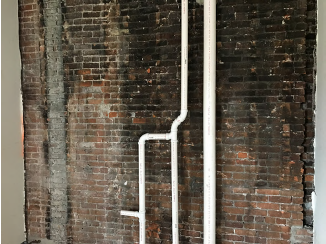
Photograph #5 – This photograph shows the wall construction at the Northern / rear of the building at the fifth floor, at the same area as Photograph #4 at the sixth floor above. This section of wall is in comparatively better shape with mortar in joints that are not dusting / disintegrating. Smoke and water staining are still present at the top of wall here but dissipates as you move down the wall. Additionally, this wall contains header brick courses about every eighth coursing which are required to tie wythes of the wall together.
