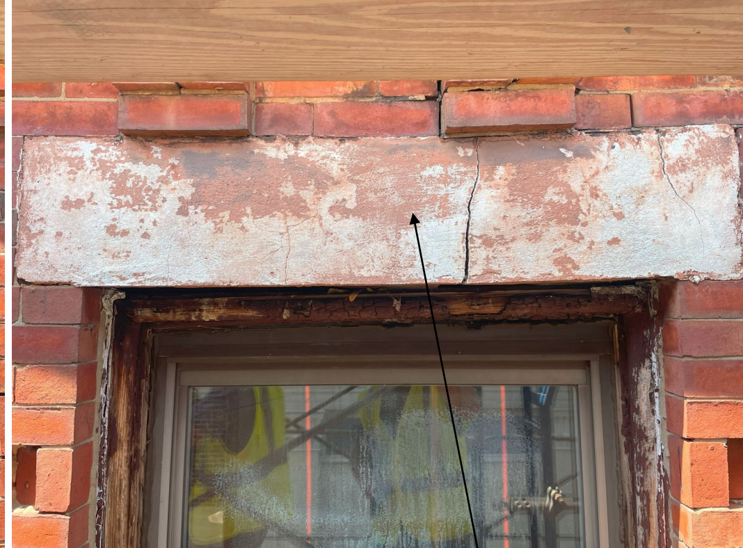
Another sagging header with non-original parging on top. Parapet corbel above has shifted due to failure of header
