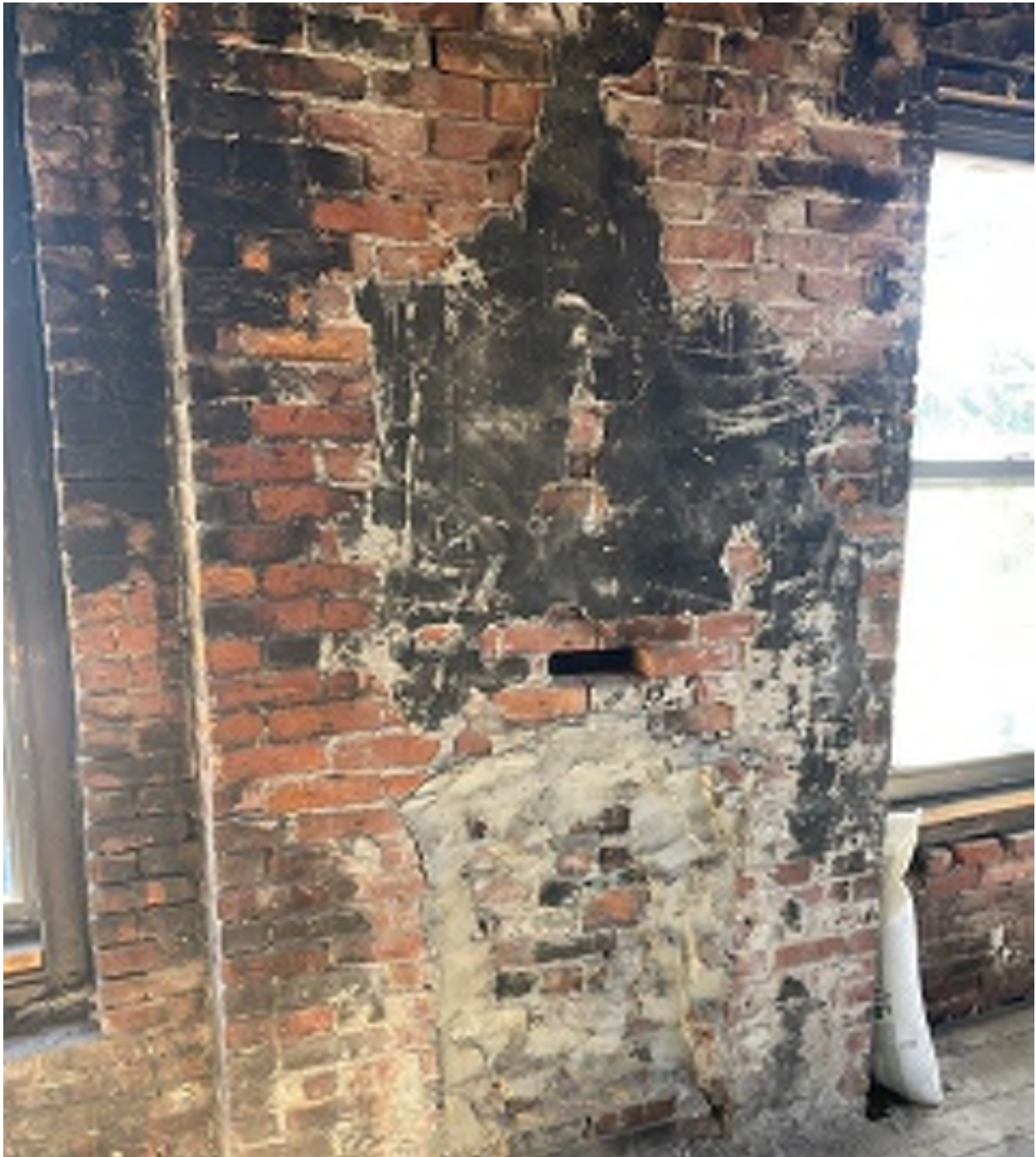
Photograph #2 – This photo shows the interior face of the existing masonry wall along Shawmut Avenue at the sixth-floor level. The masonry has receding joints, especially on the sides and below windows with dusting of mortar and loose bricks able to be removed by hand.
