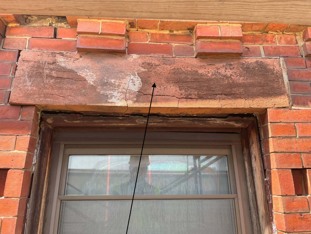
Sagging header with brick separation and window opening failures below
