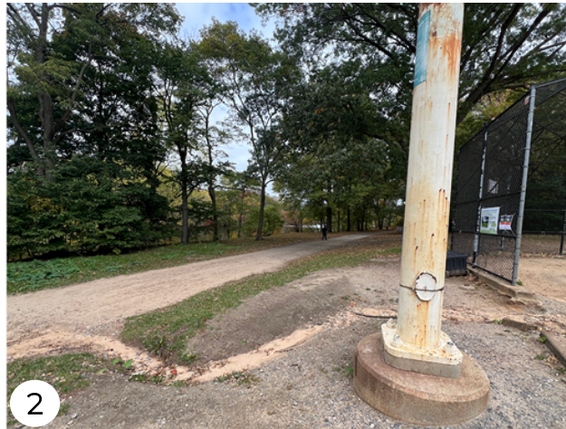
Infield mix washout from Field 1 on walkway
