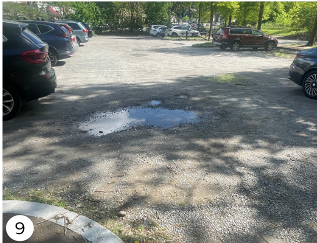
Parking Lot – Poor drainage/ponding
