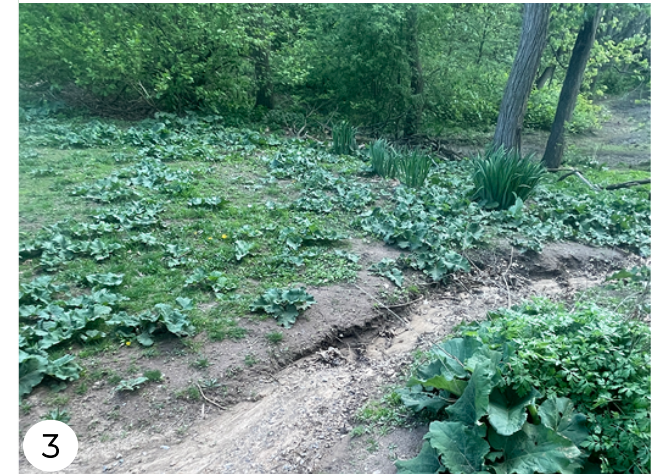
Erosion and Infield mix washout from Field 1 into pond embankment
