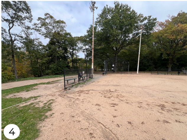
Erosion and Infield mix washout from Field 1
