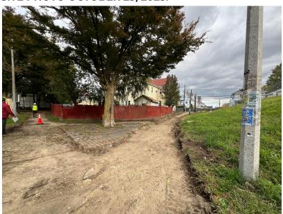
The existing concrete walkways have been demolished.
