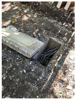
An existing electrical hand hole has been opened for inspection. Most of the existing conduit will need to be replaced.
