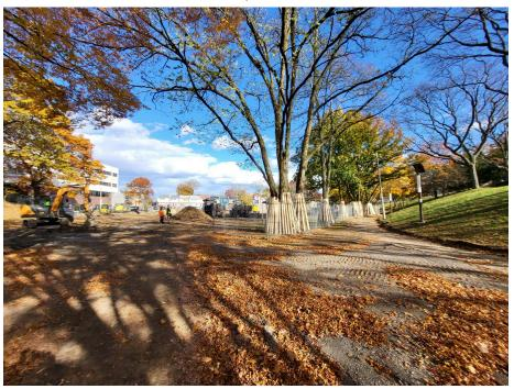
The central paving area has been demolished and the trees are being protected.
