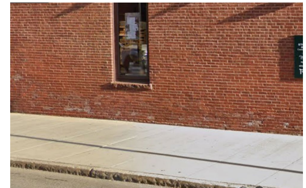
Today's corrosion and damage to base bricks on Congress St
