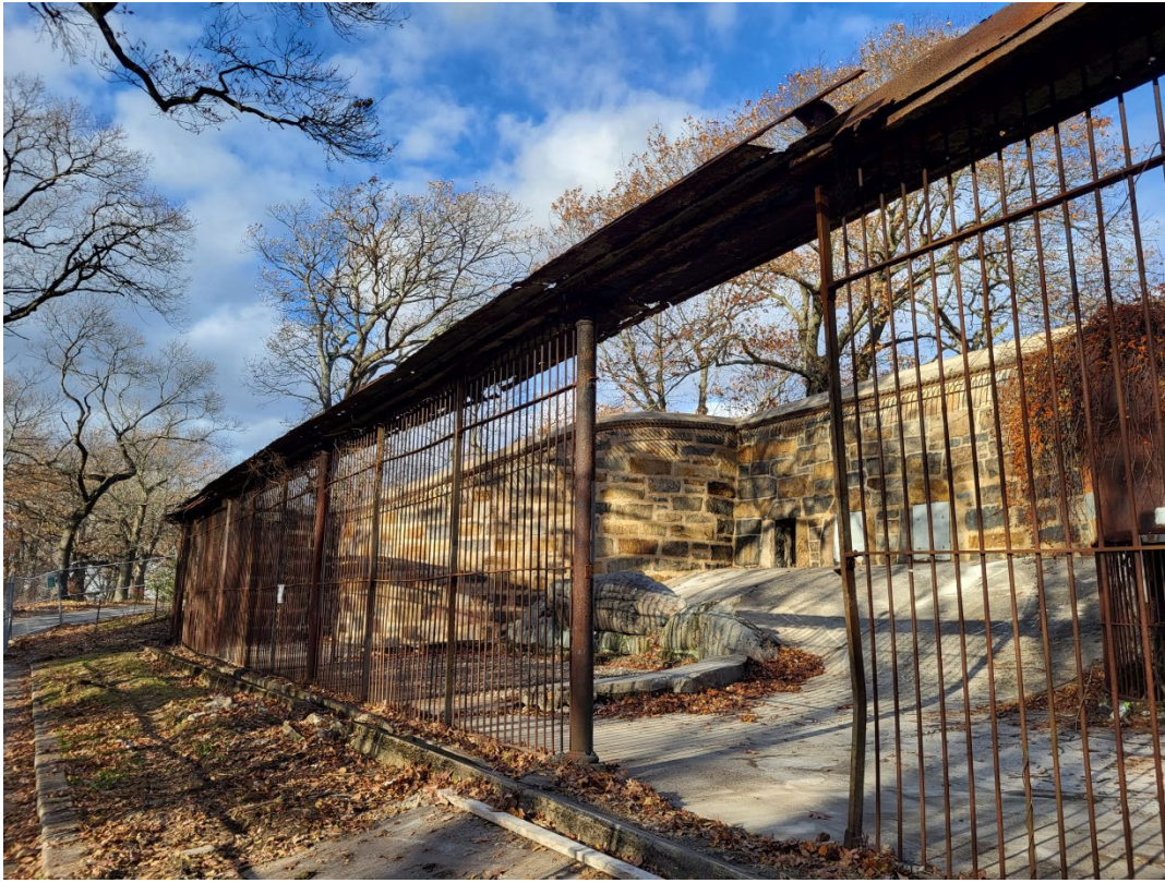
Cage 4 had the greatest amount of metal canopy remaining. The pieces will be removed and re-installed
