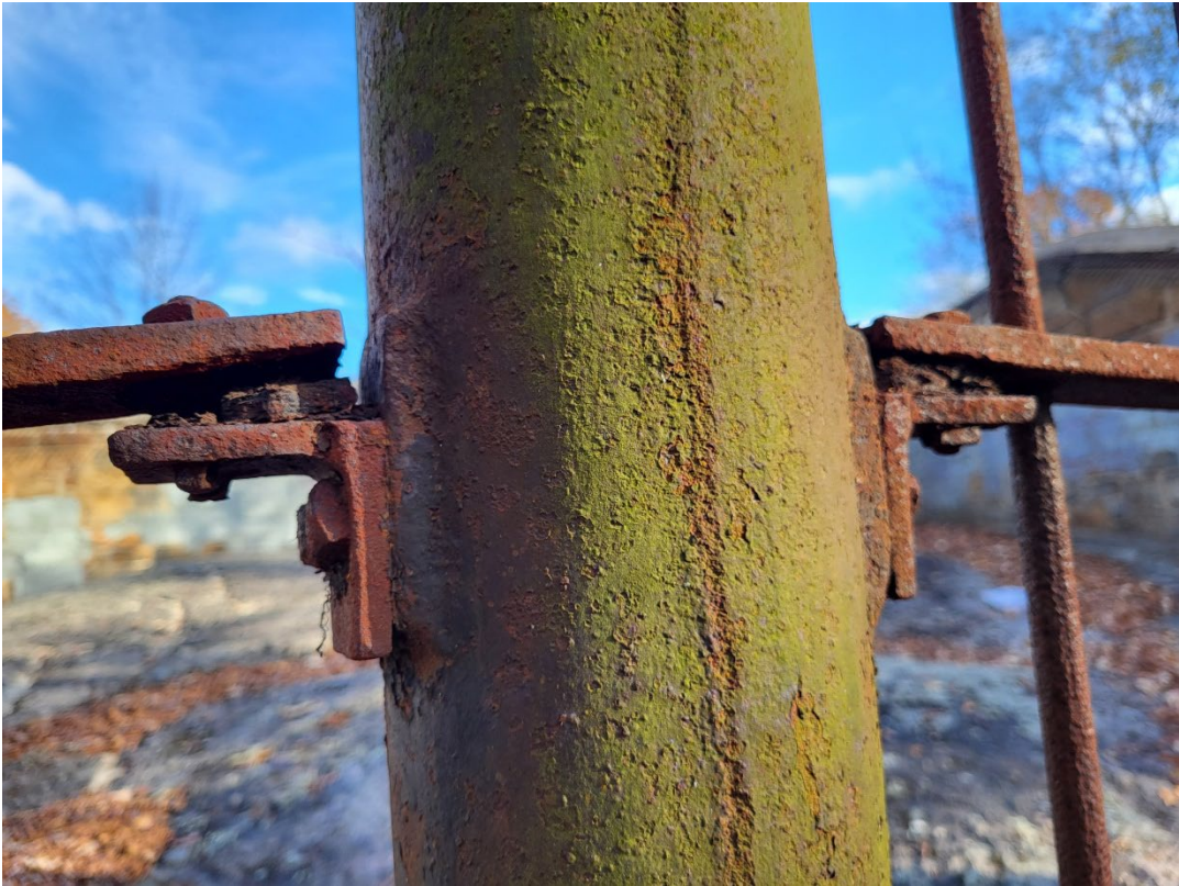
Rust has compromised the fasteners in some places. These will be reattached.
