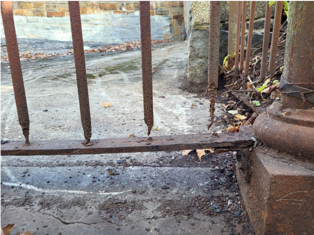
The lower portion of several pickets has deteriorated. These will be cut and installed with new metal rods.
