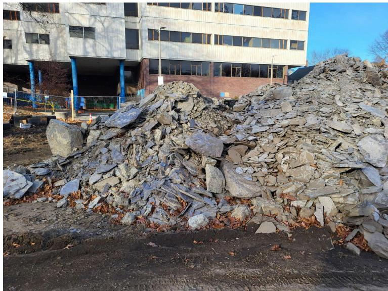
The contractor has discovered significant ledgestone beneath the site, which has added time to the construction schedule.
