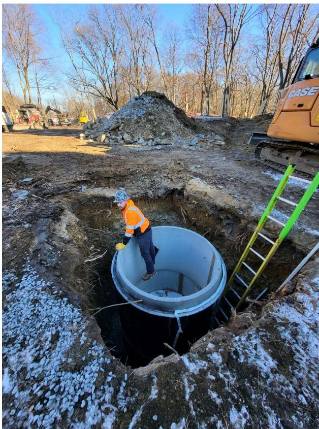
*Catch basins have been installed throughout the site. Ledgestone removal was required for this installation.*
