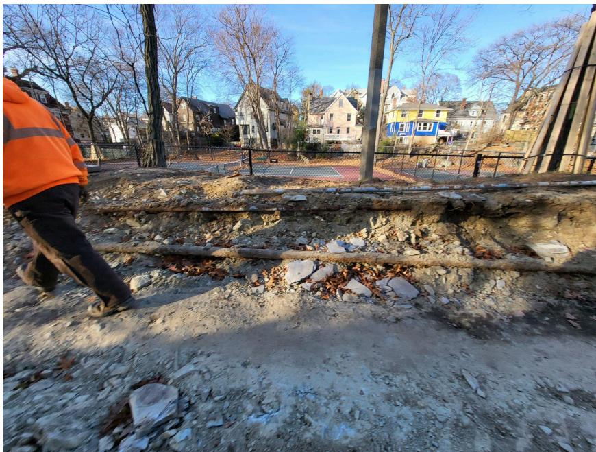
*The existing electrical conduit is higher in elevation and in poorer condition than anticipated; it will need to be replaced.*
