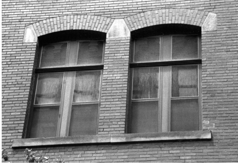
Fig. 21. Stilted arches, formed of a segmental arch with contrasting stilts at the springing line. Photograph of 34-46 Farnsworth Street.
