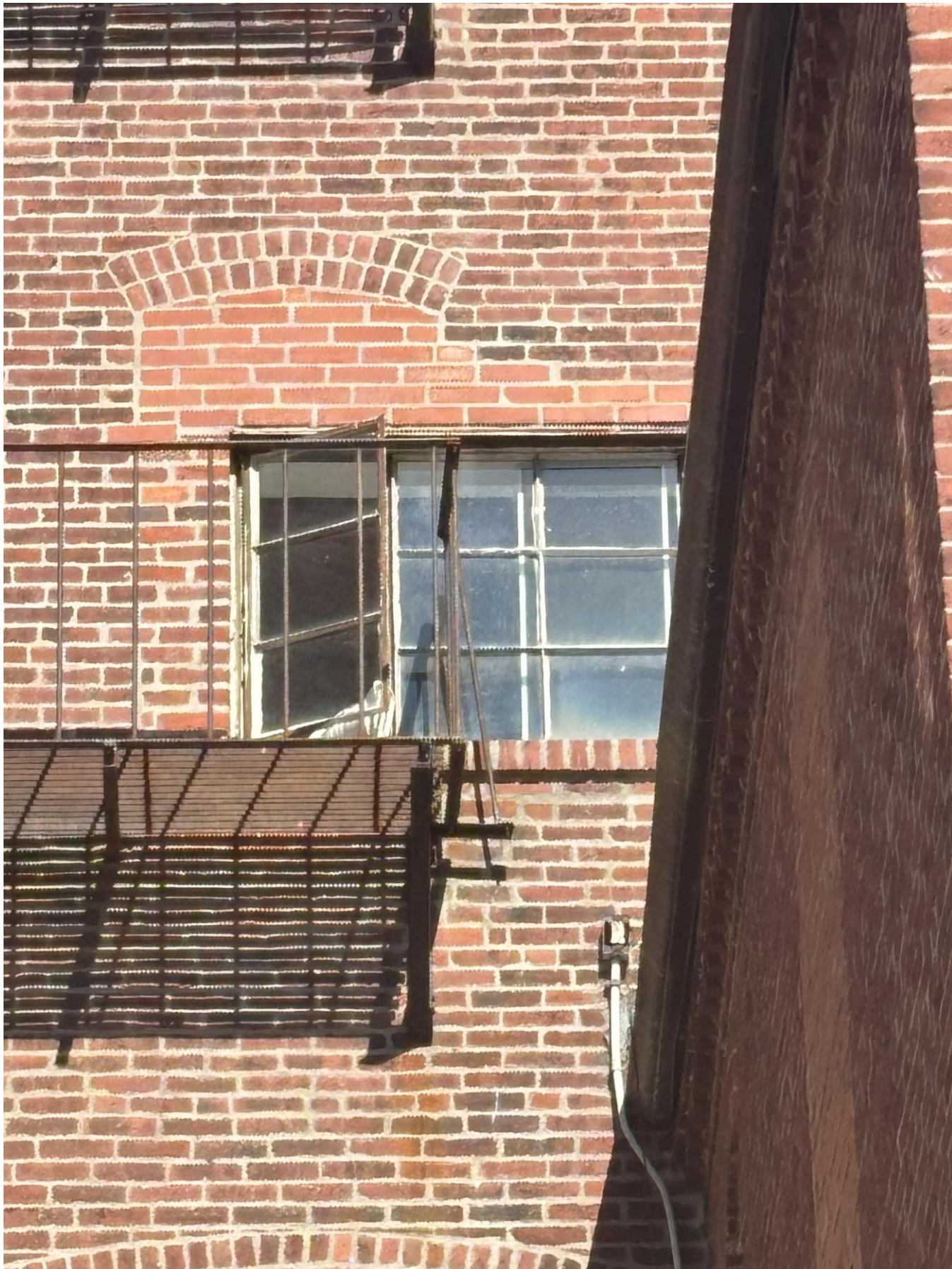
REAR ELEVATION – CLOSE UP OF THE ONE WINDOW TO BE REPLACED
