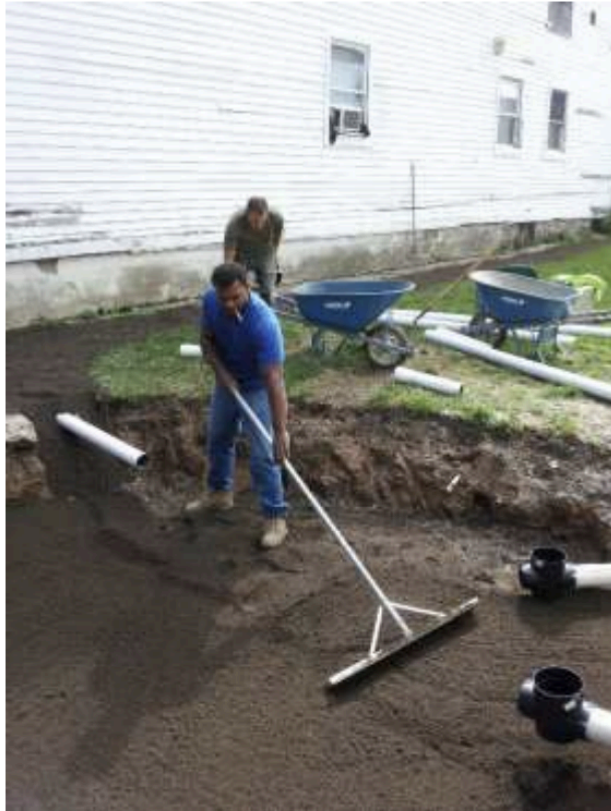
PUSH Blue crew working on green infrastructure in Buffalo's west side
