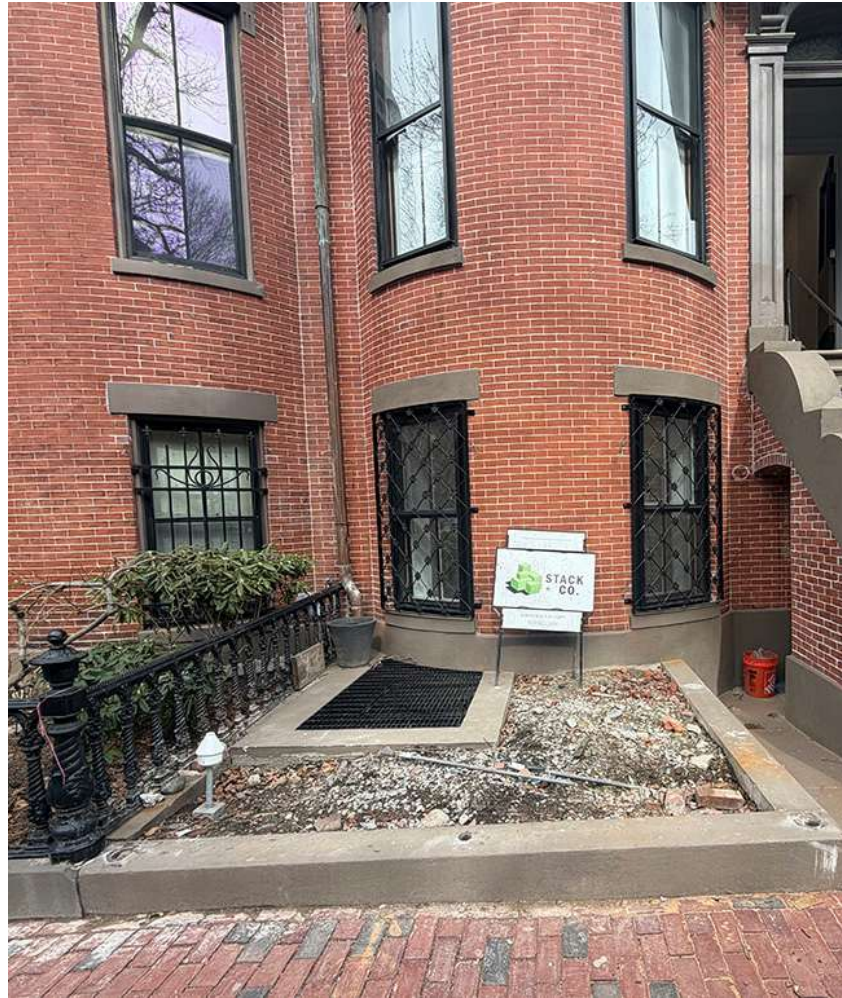
Unapproved garden fence removed
