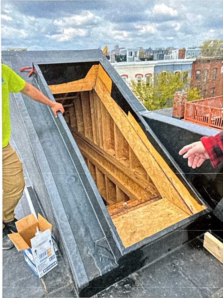
19 W. Cedar St Roof Access Hatch & Rough Framing Example
