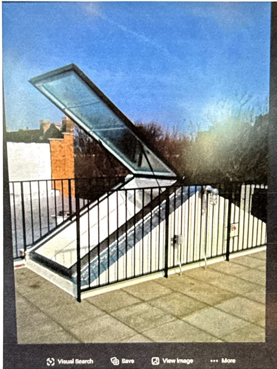
19 W. Cedar St Roof Access Hatch 3 Installed Example
