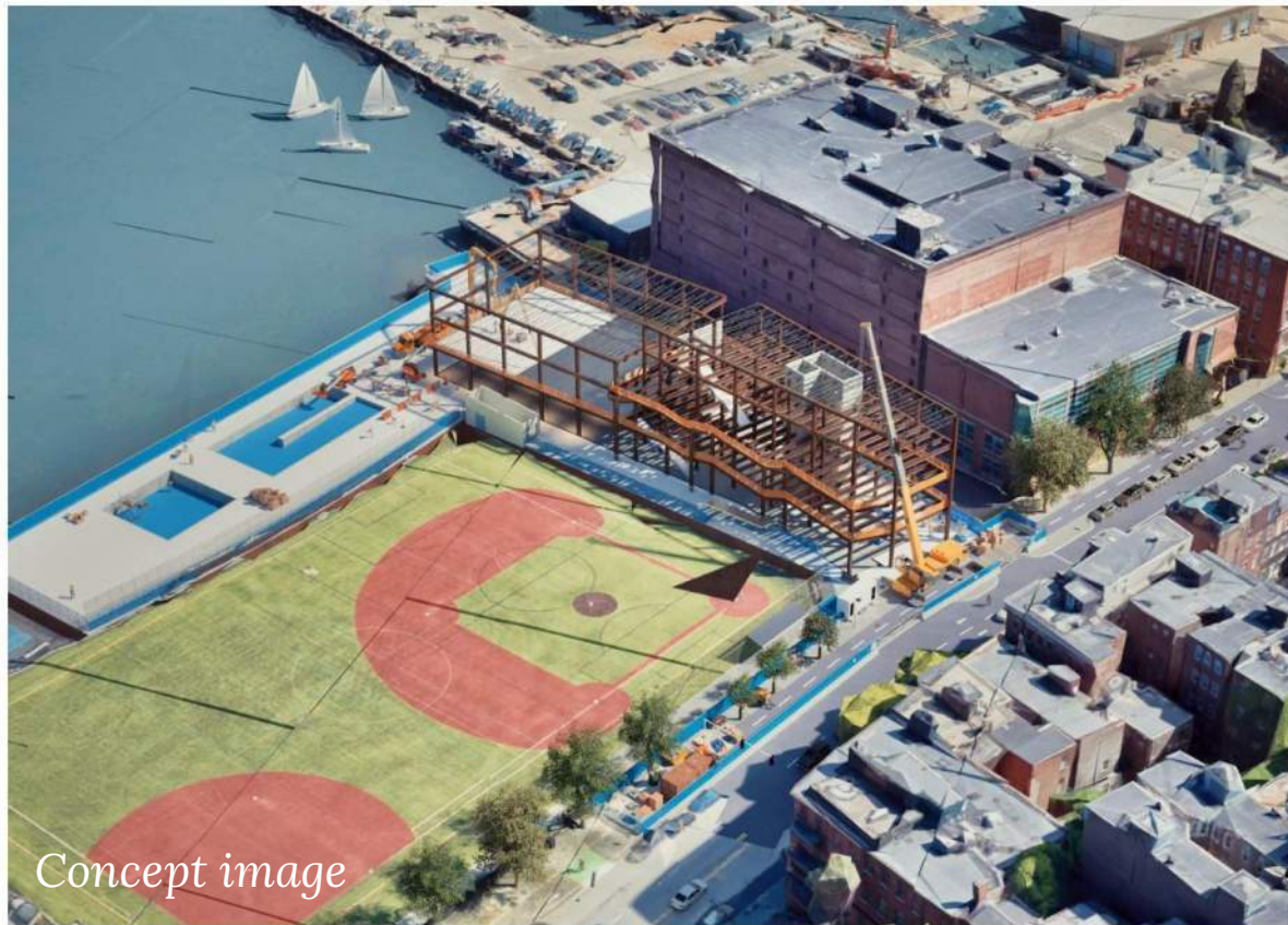
North End Community Center Structural Steel
