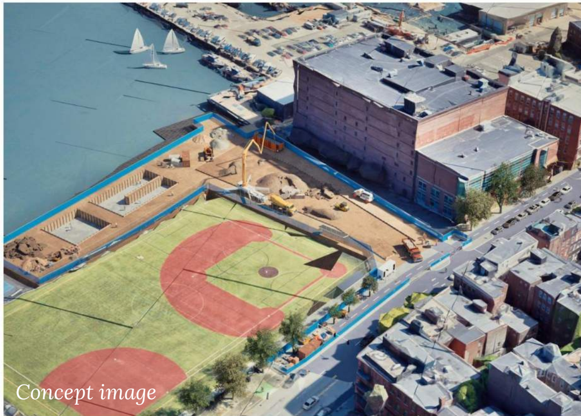
North End Community Center Excavation
