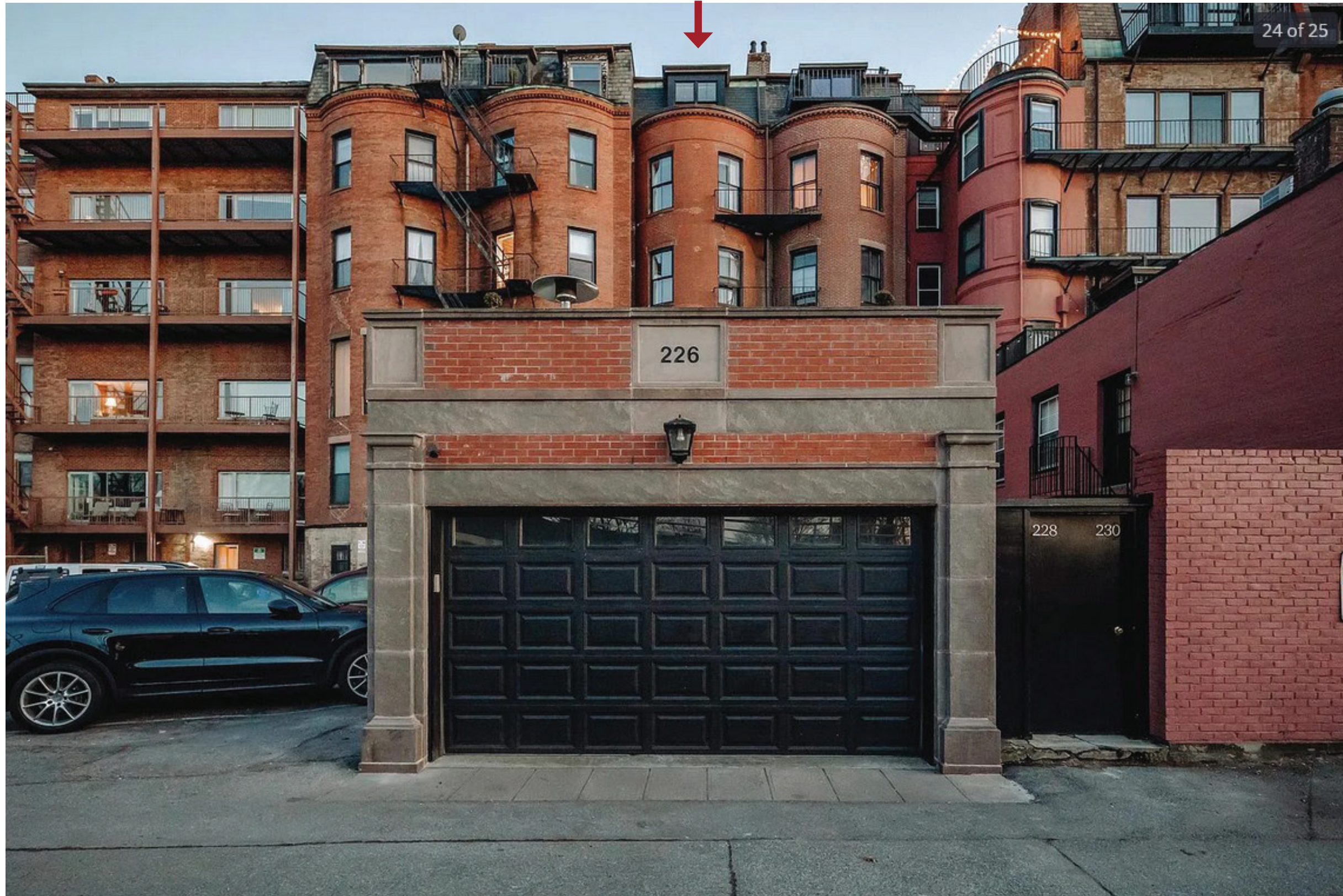
Existing Rear Facade and Garage Door Garage and Terrace constructed ca. 2011
