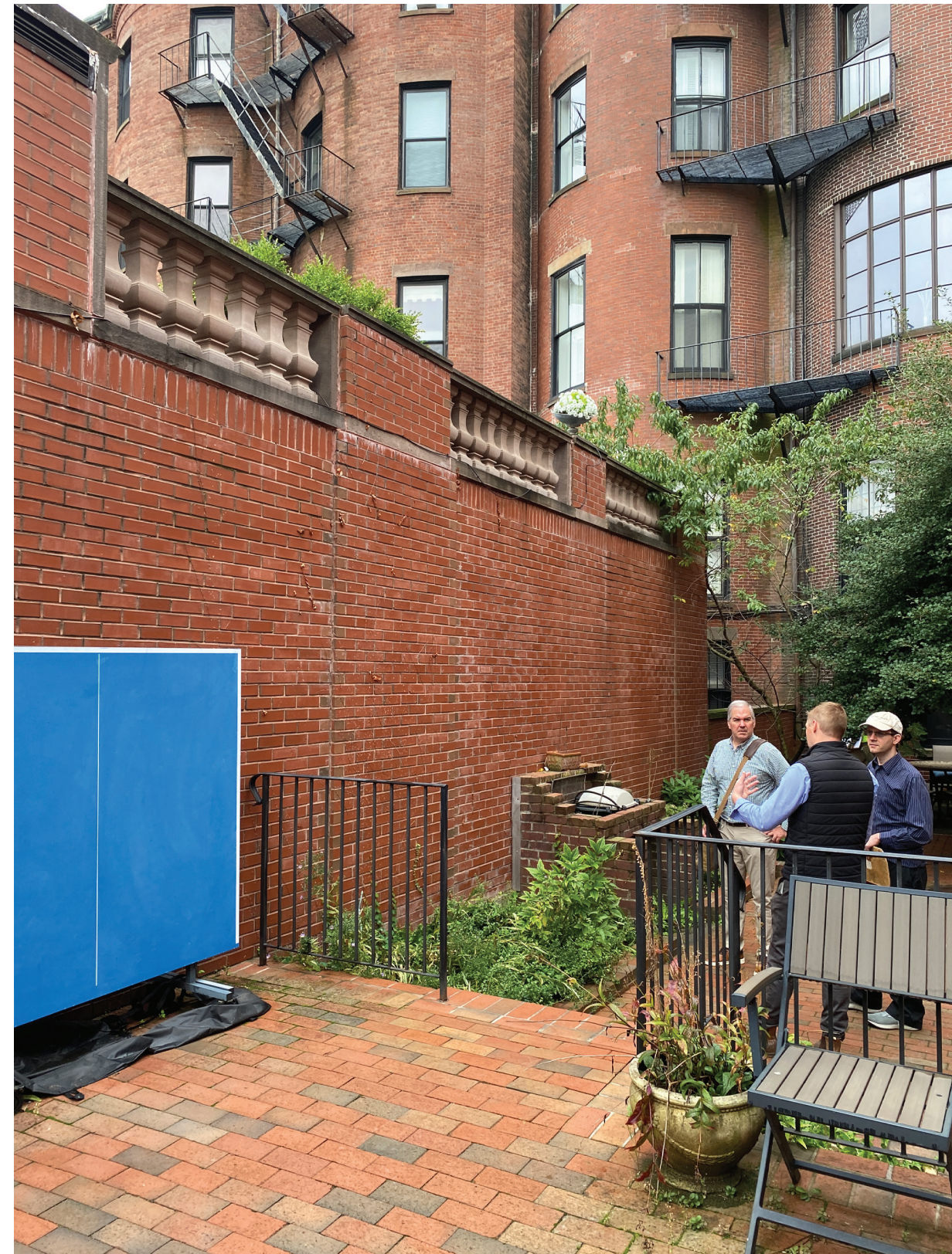
Existing West Facade Garage and Terrace constructed ca. 2011
