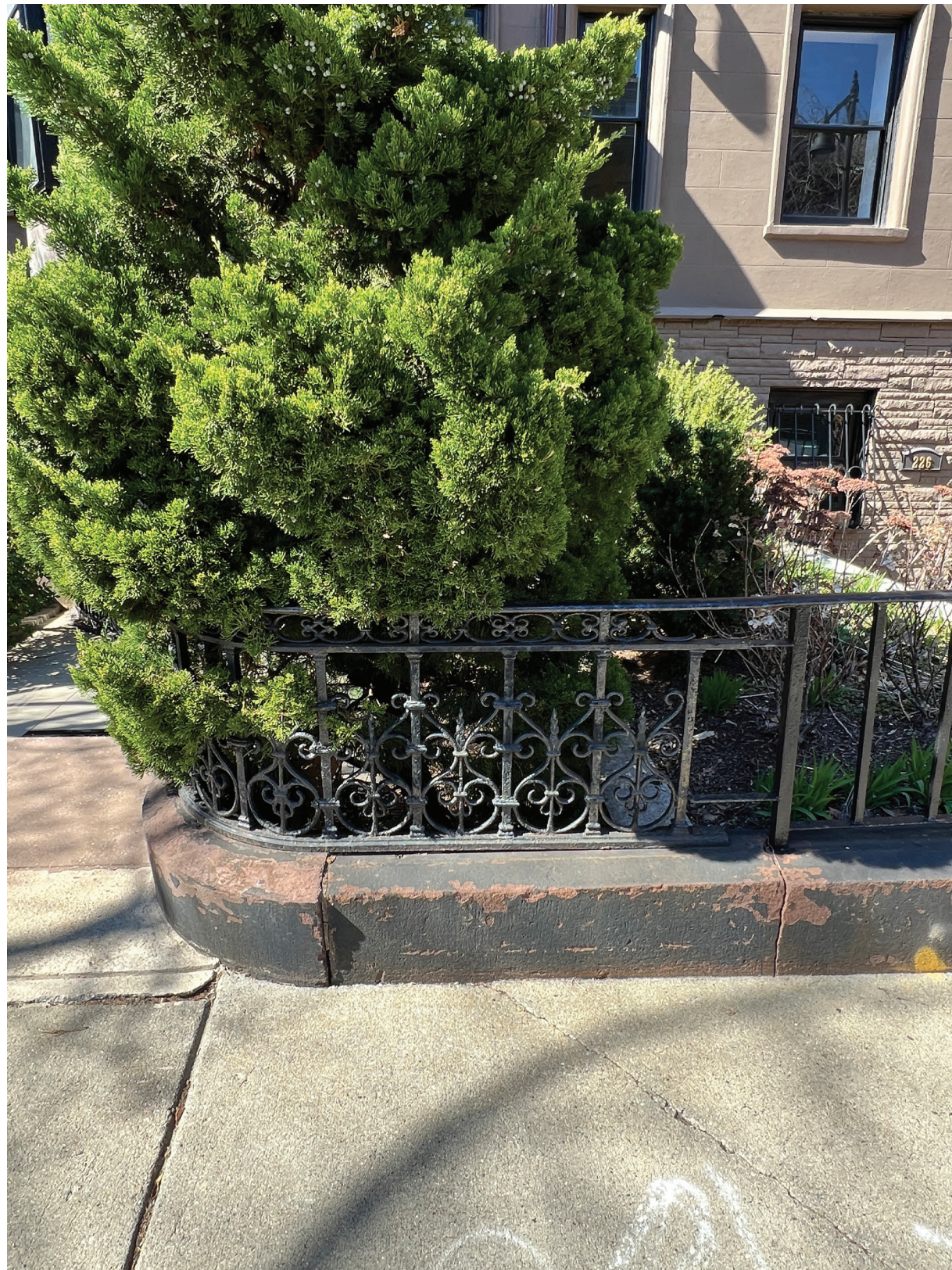
Existing Historic Fence at Neighboring Property
