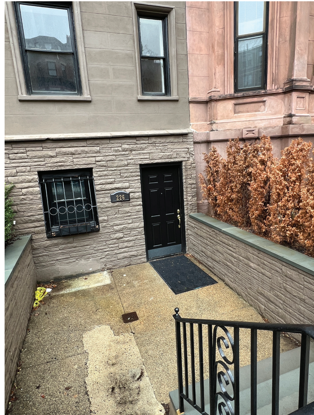
Existing Sunken Courtyard and Basement Entrance
