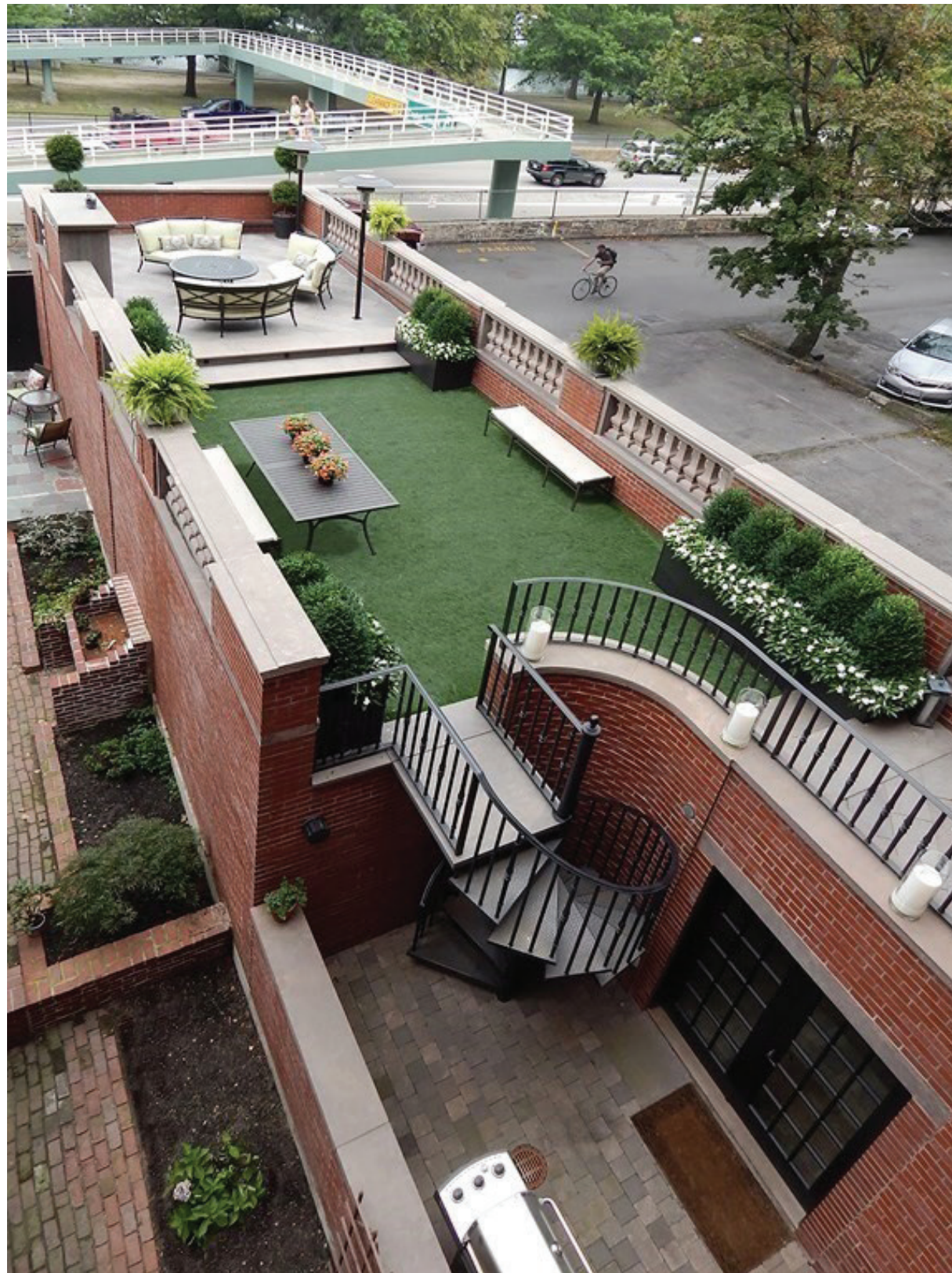
April 2025 - Condition of Rear Terrace
