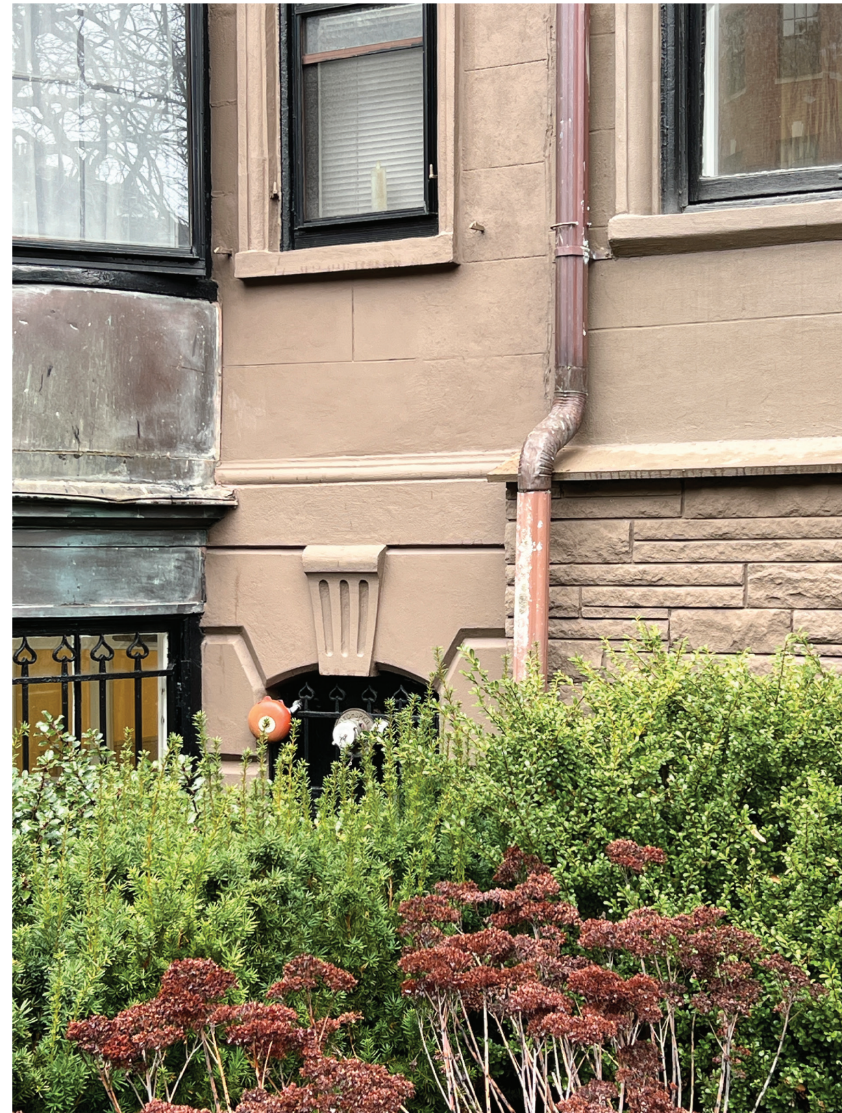
Existing Applied Rock Face Veneer Next to Historic Stonework at Neighboring Property
