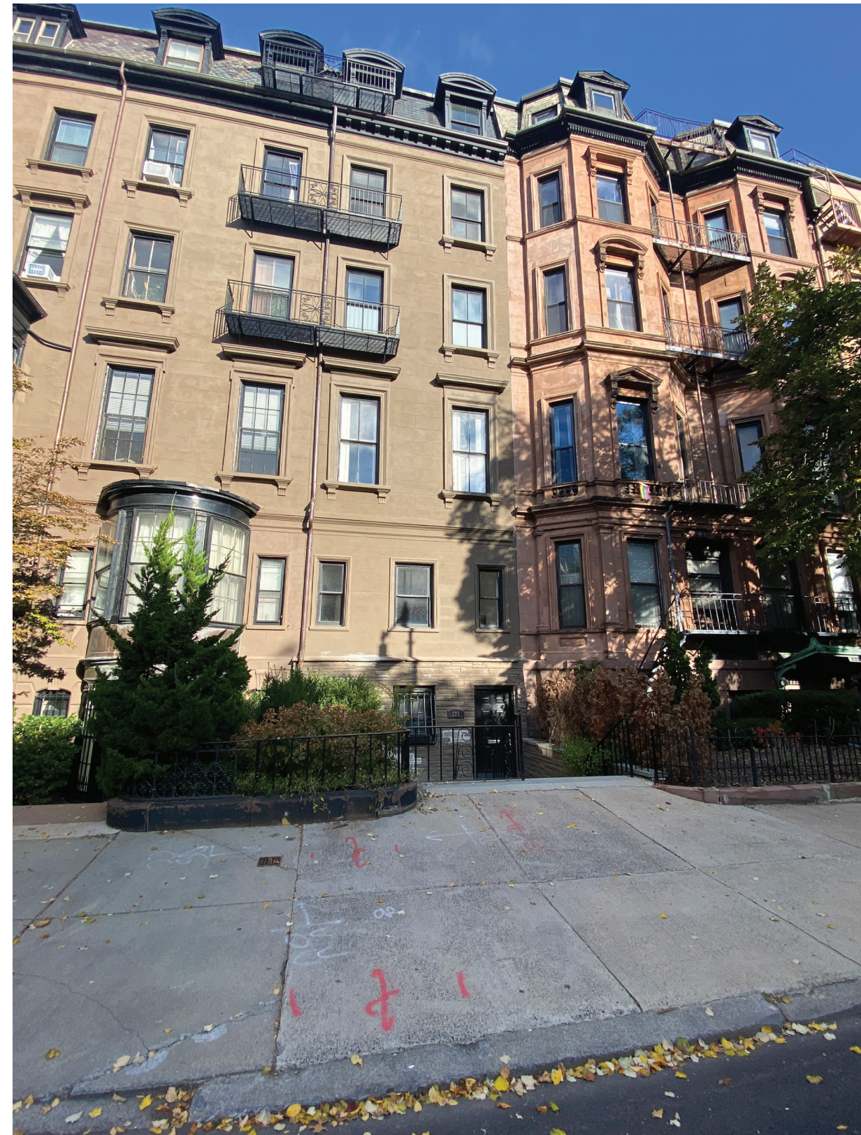
Existing View At Sidewalk
