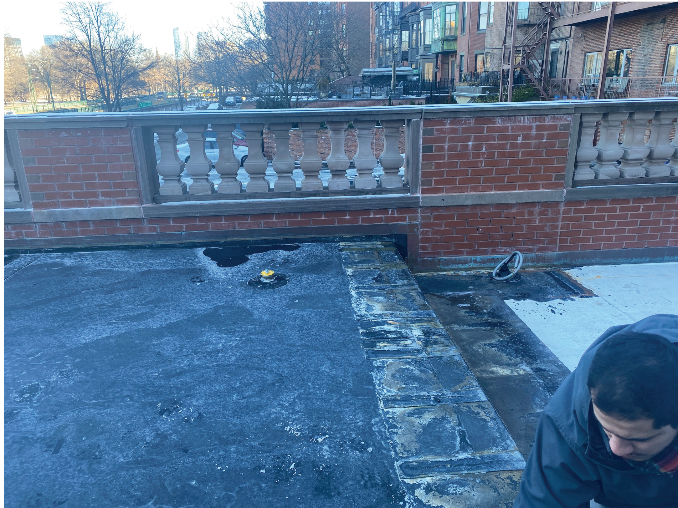
January 2026 - Existing Brick and Stone Terrace Walls
