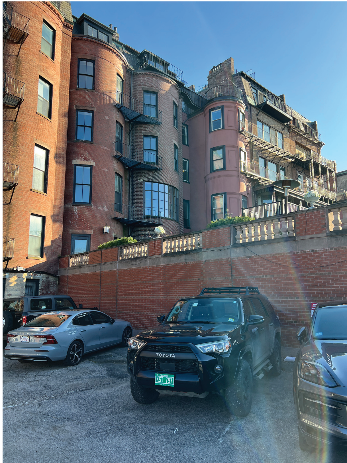
Existing East Facade Garage and Terrace constructed ca. 2011
