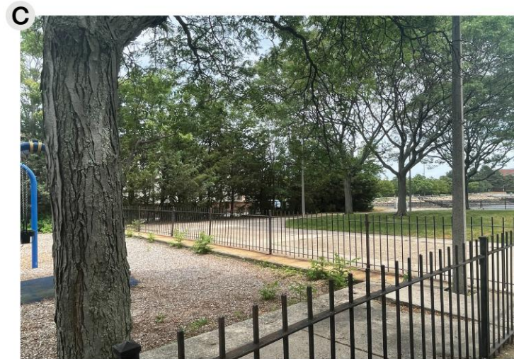
C Playground Fencing
