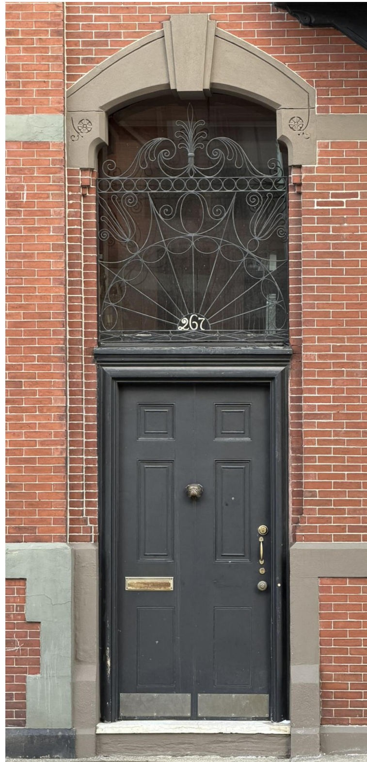
267 Clarendon Street, Existing Door
