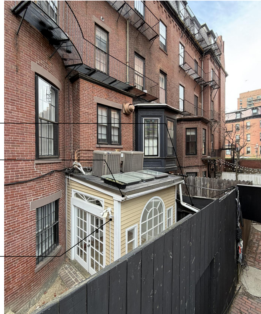
Existing Rear Addition
