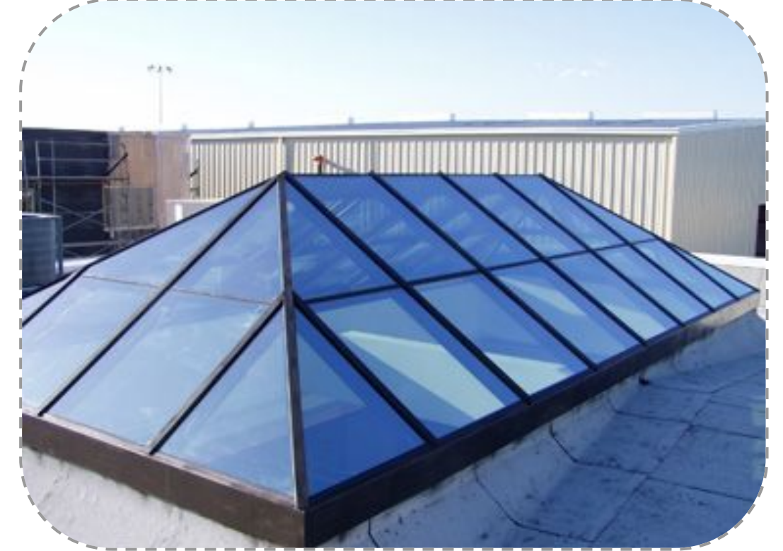
Example of similar skylight.
