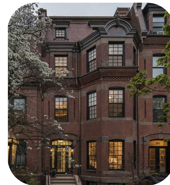
Example of new windows at 320 Marlborough Street
