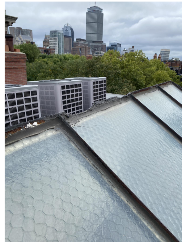
Existing skylight, showing failing glazing putty and corrosion at joints.
