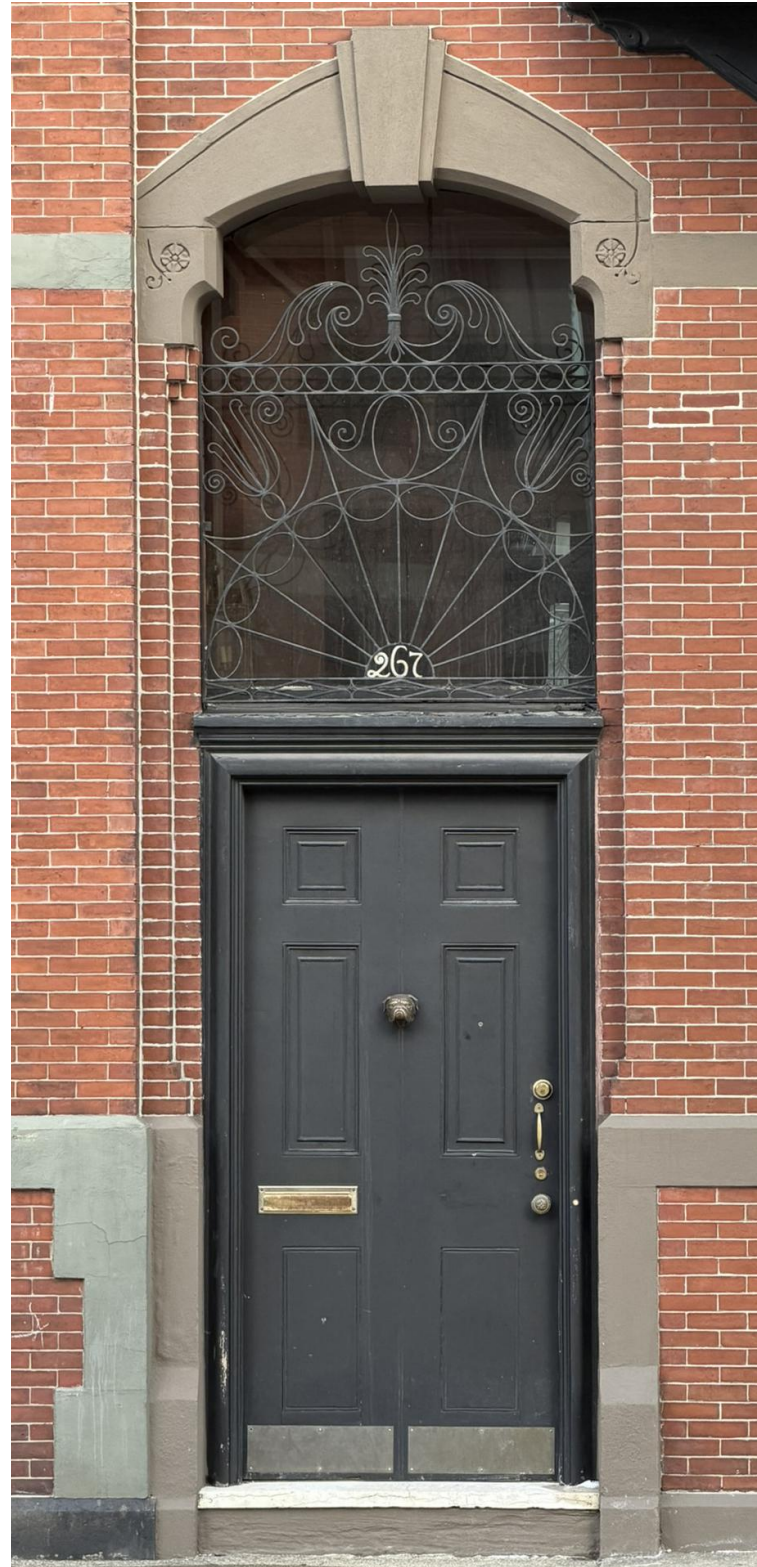
267 Clarendon Street, Existing Door
