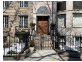
Remove Existing Gate at Main Entrance
