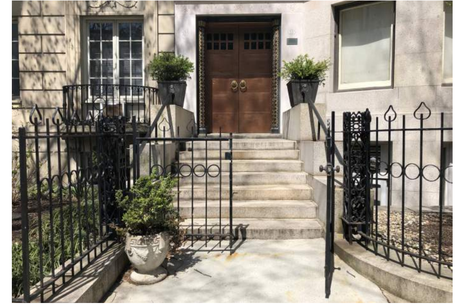
Existing Fence and Gate
