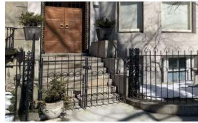
Keep Existing Handrails at Main Entrance
