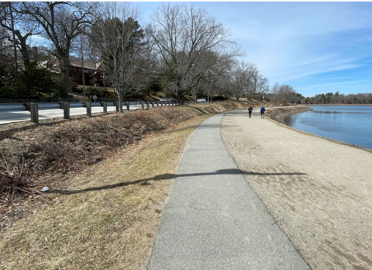
View northwest showing existing conditions at proposed location of oval planting bed to left of paved pathway.
