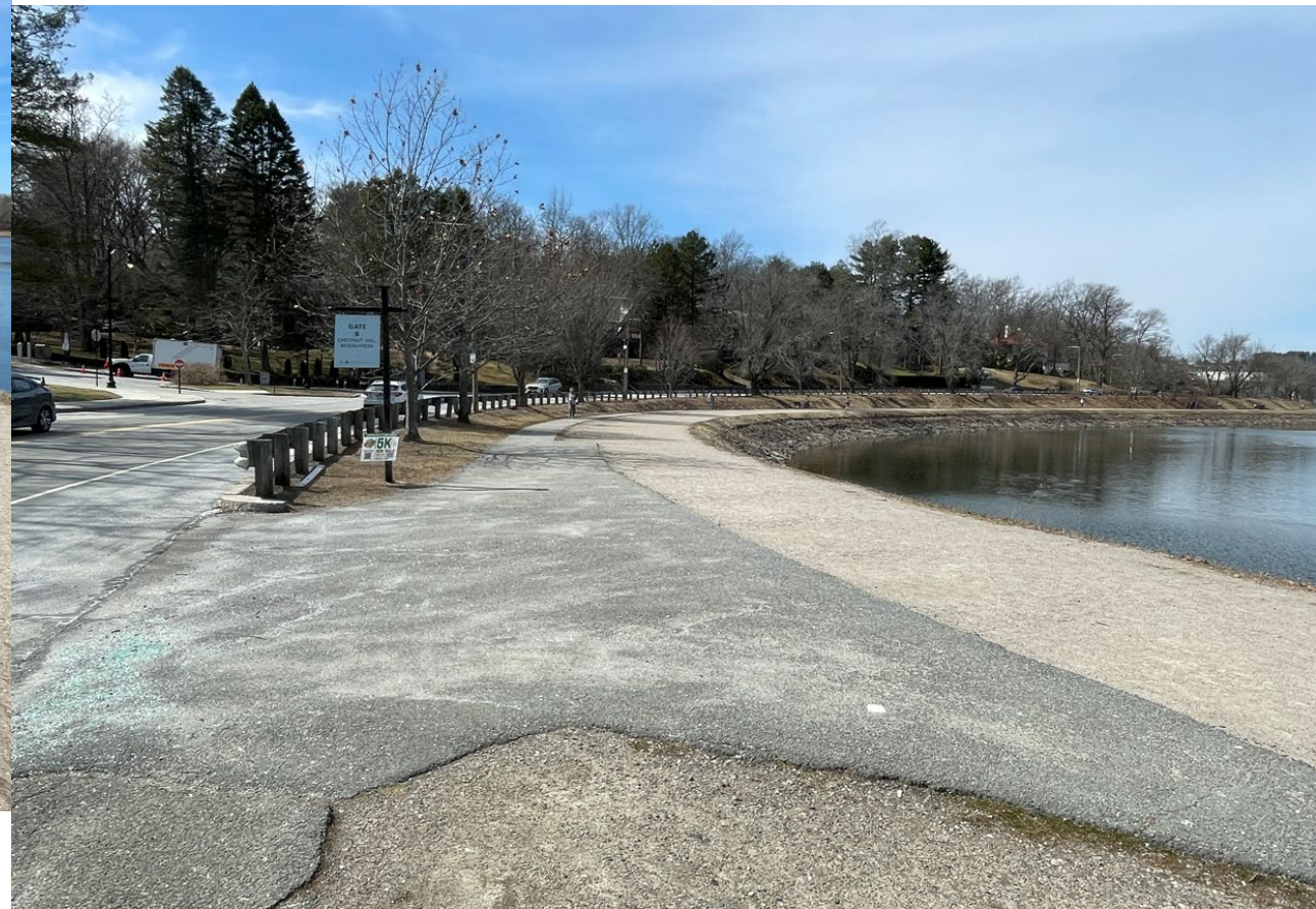
View west from southern terminus of project area.
