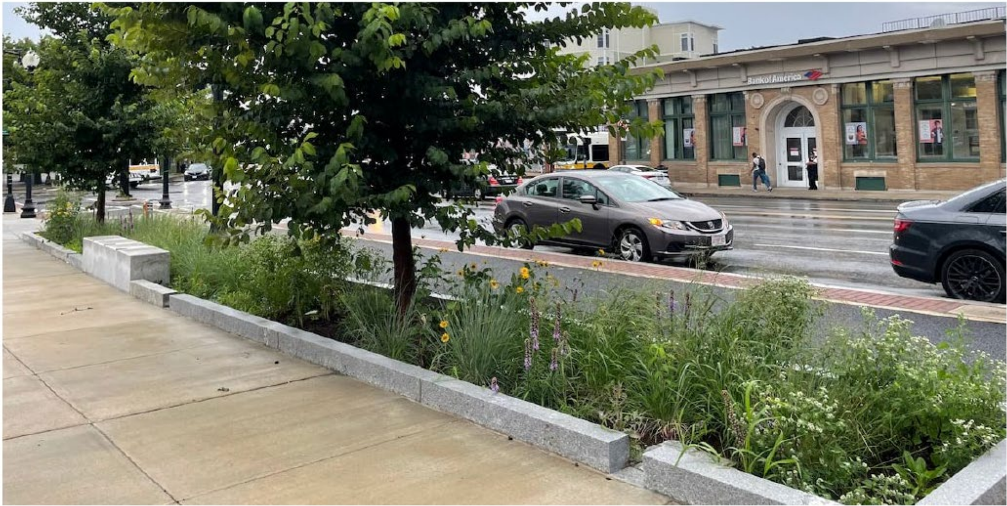
View of bioretention swale with granite curbs and weirs installed at 114 Dudley Street in Roxbury as example of similar installation proposed for Chestnut Hill Reservoir (minus trees).
