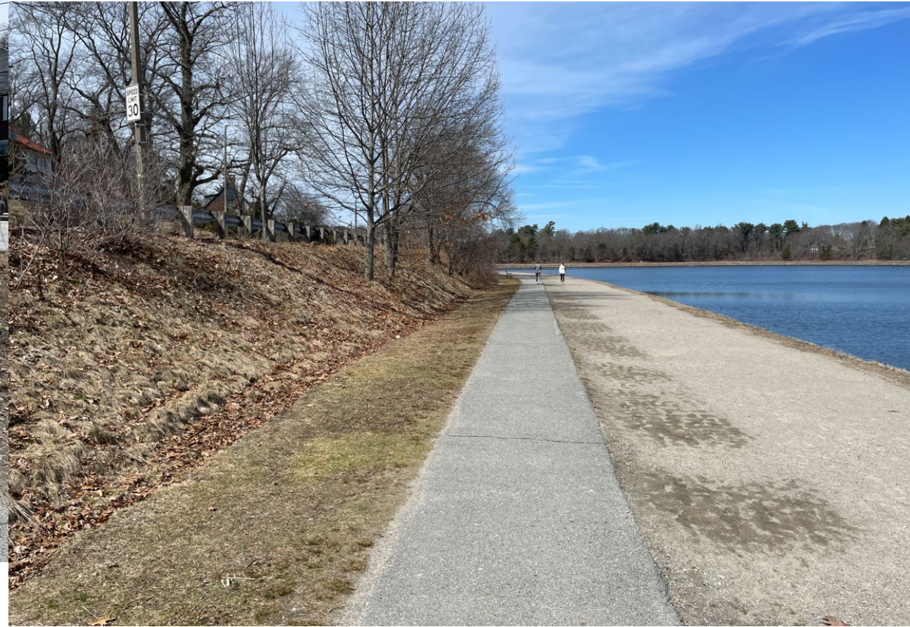
View northwest along southern half of project area showing typical existing conditions.
