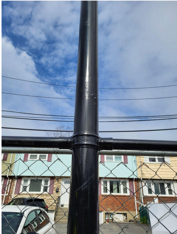
The ballfield posts will be refurbished.
