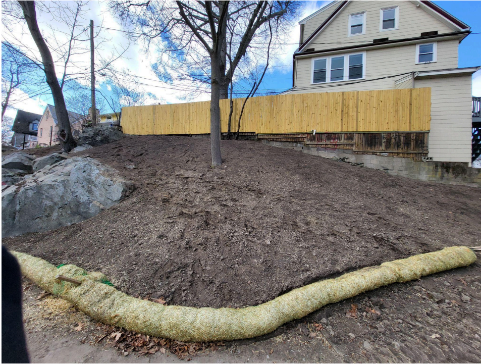
Part of the perimeter chain link fence that was not necessary was removed.
