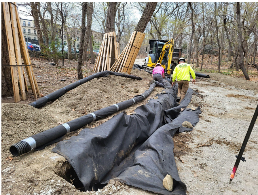
Drainage infrastructure getting laid along the woodland path.
