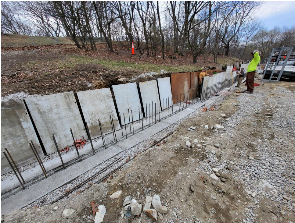
The reinforcement for the concrete site walls has been placed.
