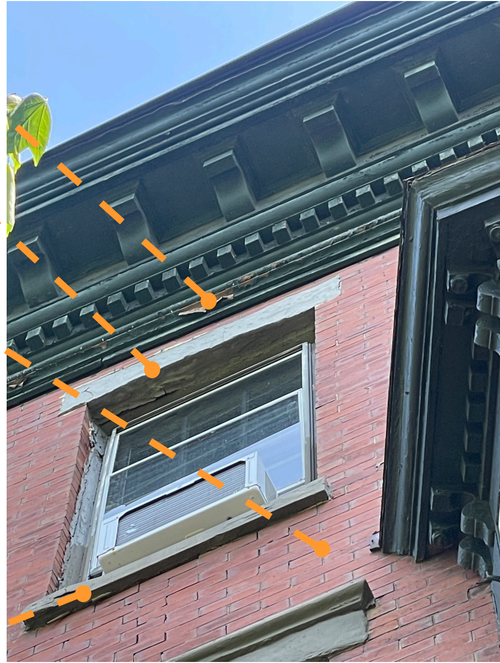
139 WEST CANTON - FOURTH FLOOR WINDOWS
