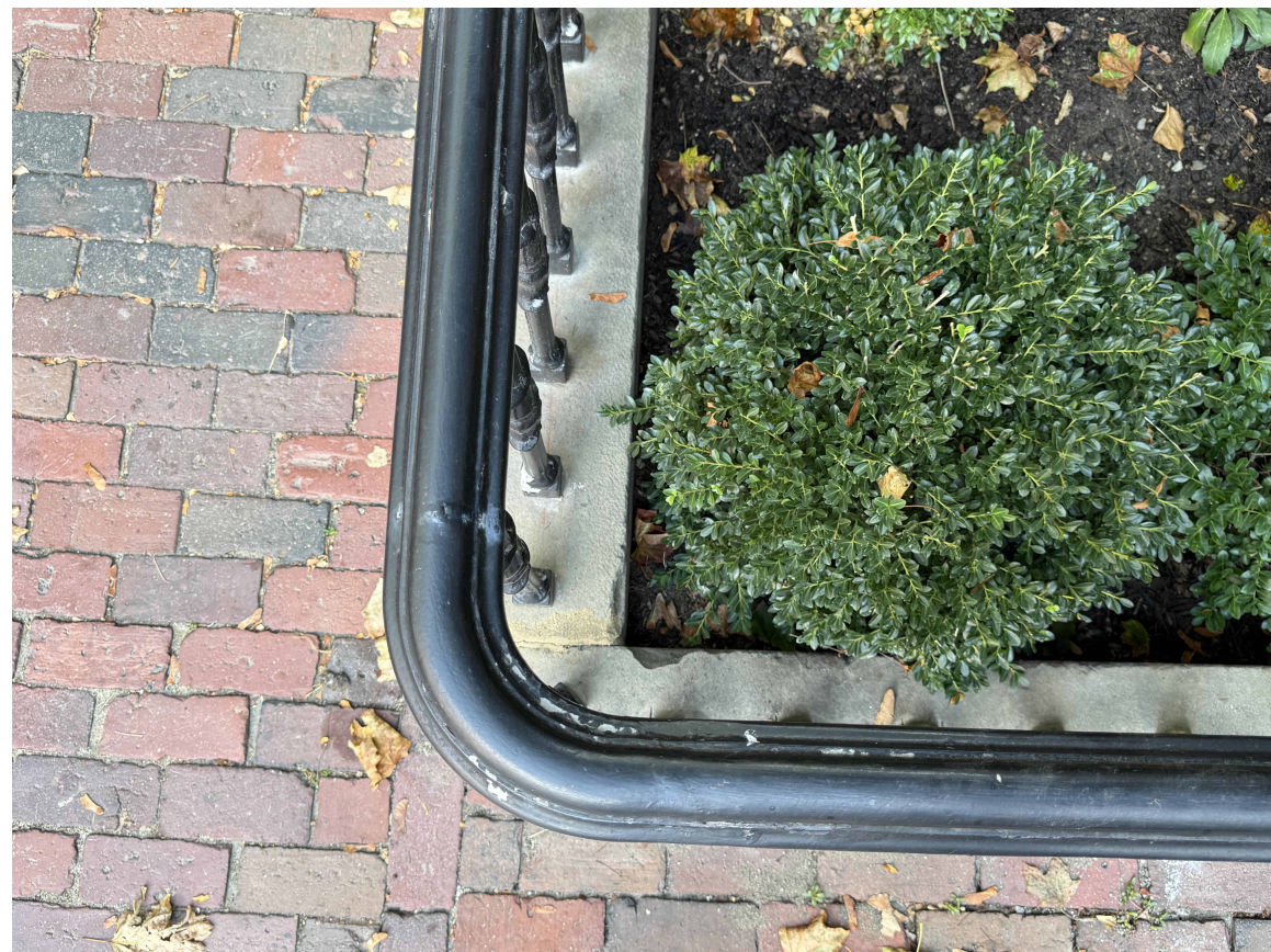
North Fence Corner to be Model for New Corner
