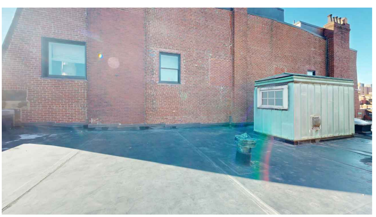
EXISTING HEADHOUSE ALONG WEST PARTY WALL
