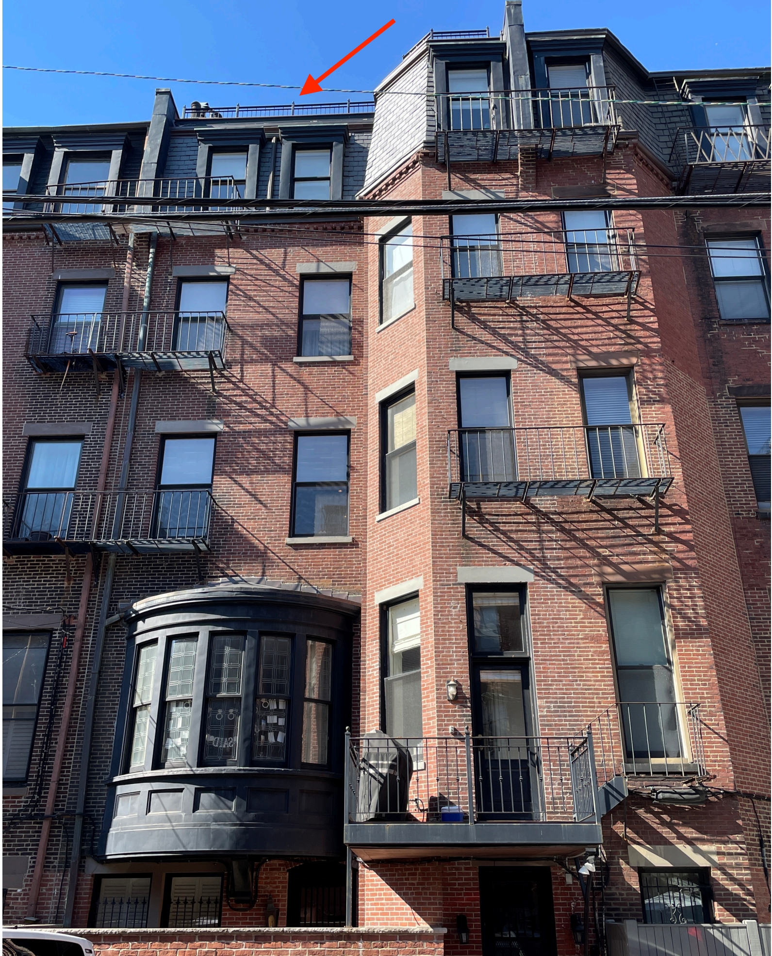
Rear Deck Existing Conditions
