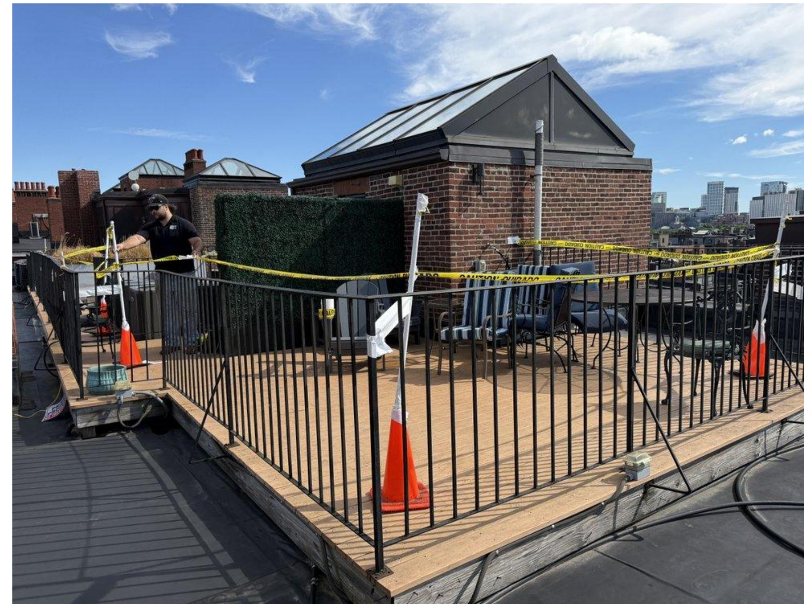
YELLOW RIBBON MOCKUP INDICATES PROPOSED RAILING LOCATION.
