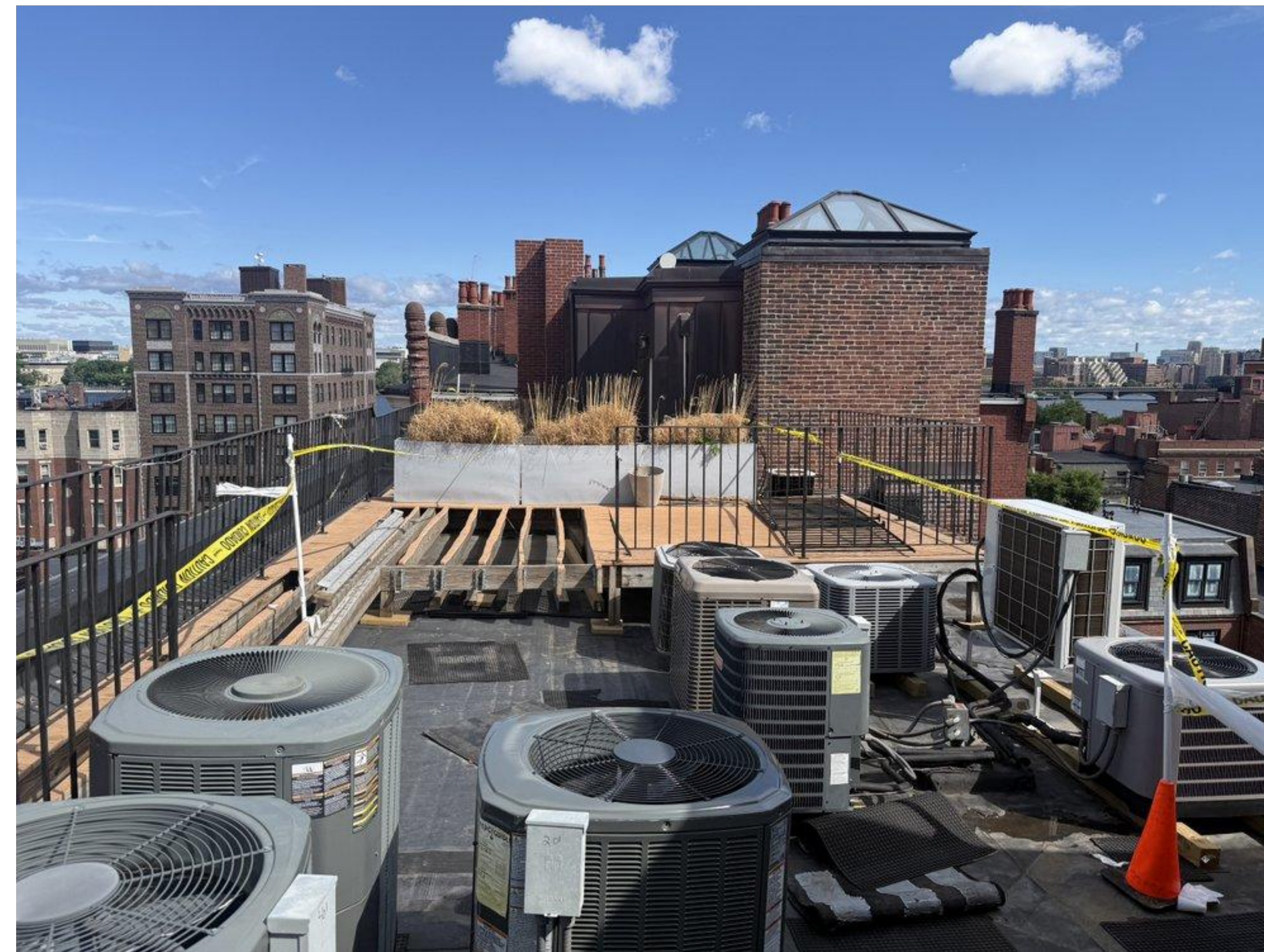
YELLOW RIBBON MOCKUP INDICATES PROPOSED RAILING LOCATION.
