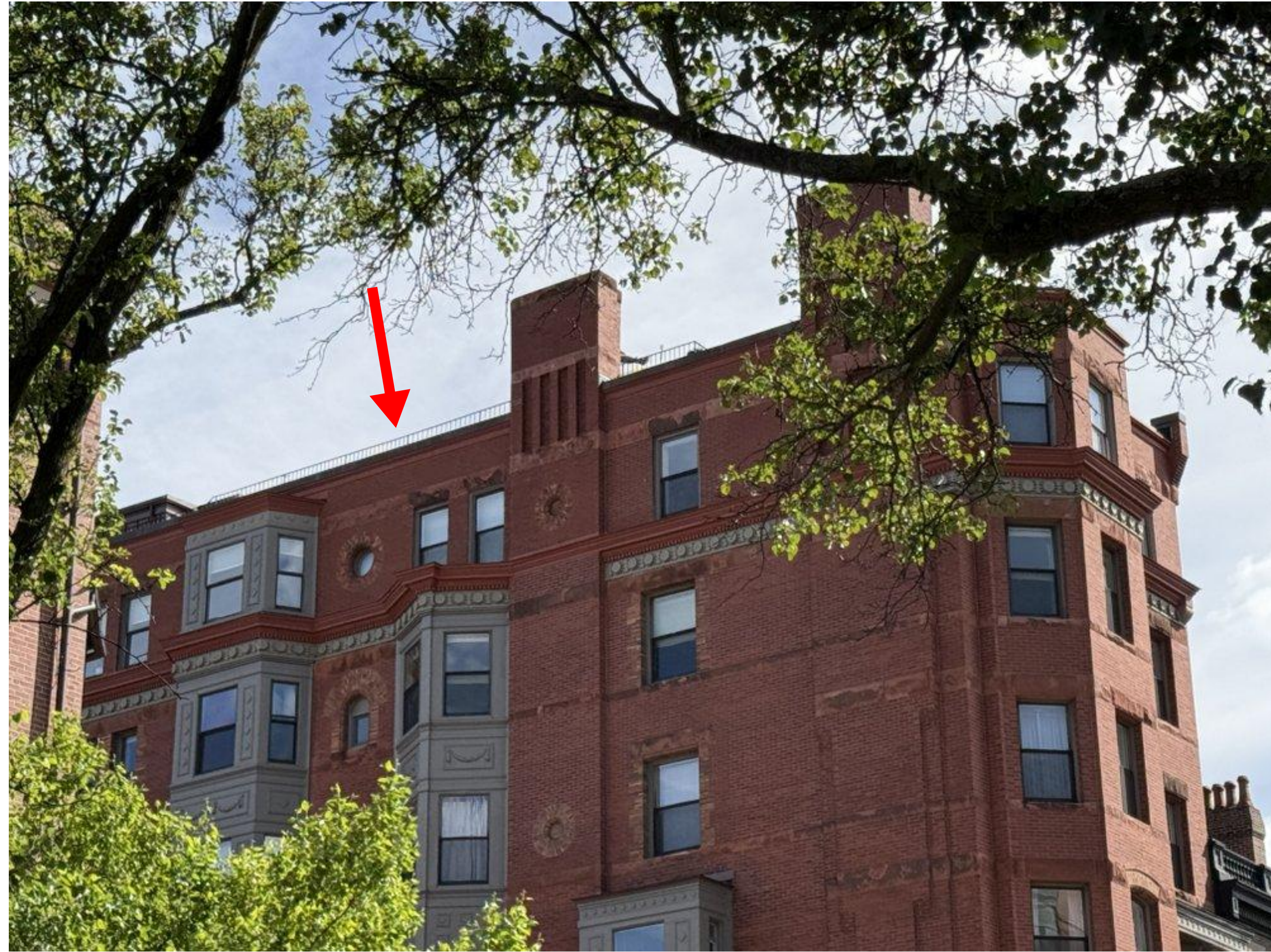
ZOOMED IN VIEW FROM MARLBOROUGH STREET LOOKING WEST - MOCKUP RAILING IS NOT VISIBLE
