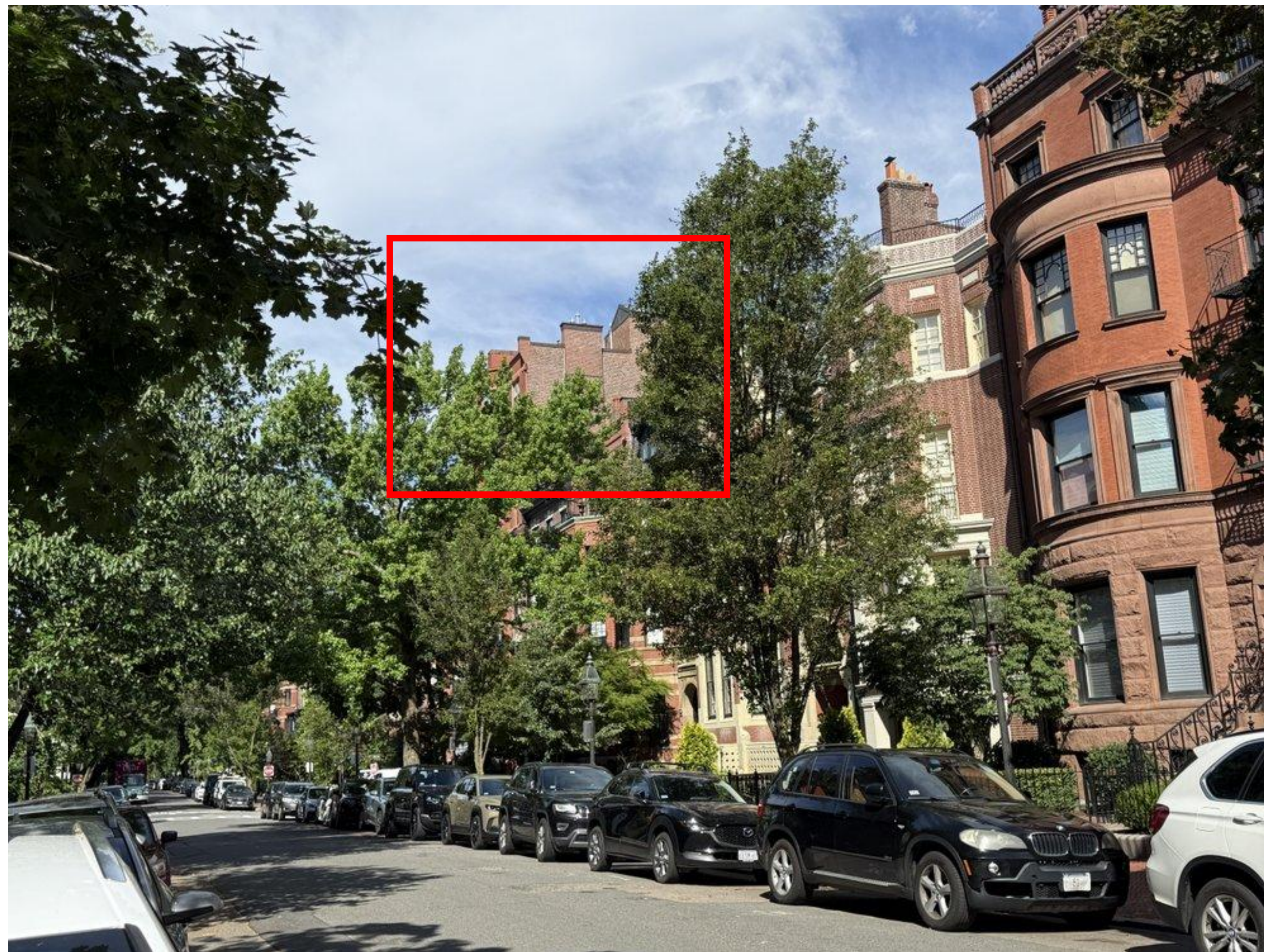
STREET VIEW FROM MARLBOROUGH STREET LOOKING EAST - MOCKUP RAILING IS NOT VISIBLE
