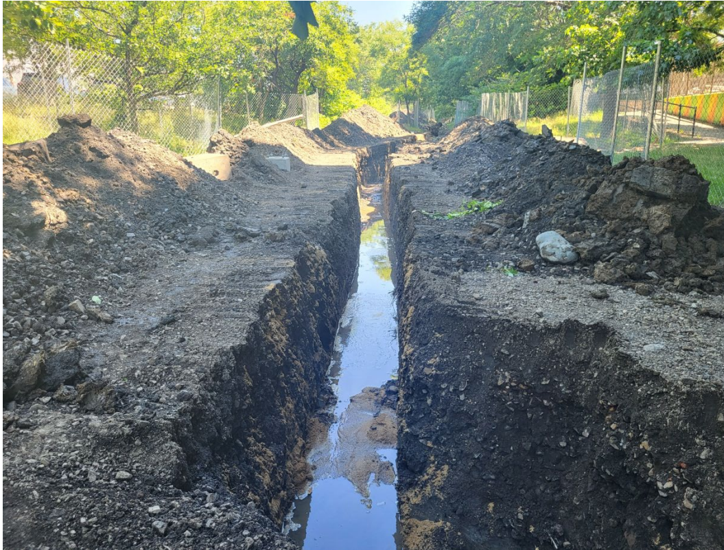
A trench for the new water line filled with several inches of groundwater (above), the existing water vault (below left) and shells in the excavated material (below right)
