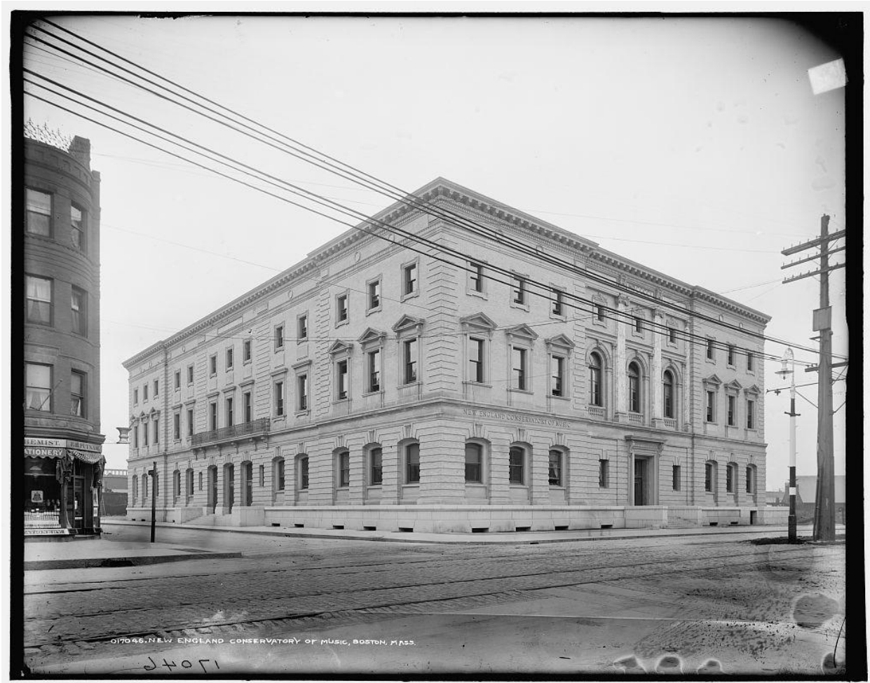
Figure 24. New England Conservatory original building, photograph circa 1904. 2
