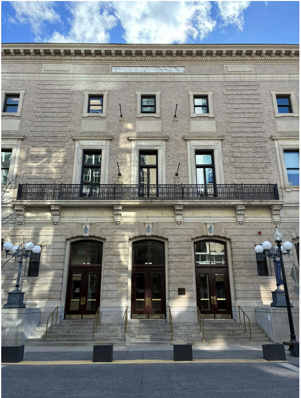
Figure 15. Detail of entrance on Gainsborough Street. March 2026 by Jennifer Gaugler.
