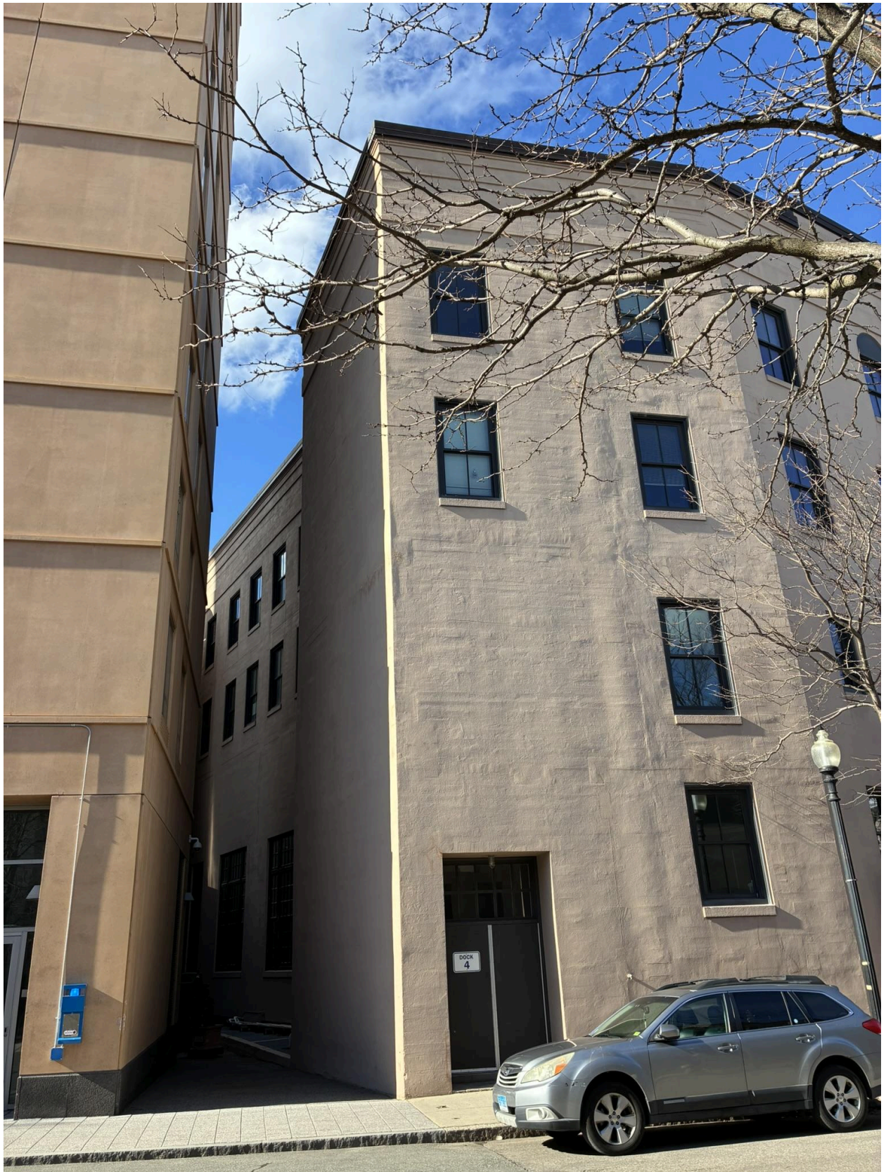
Figure 19. Facade of later addition (Brown Hall). March 2026 by Jennifer Gaugler.
