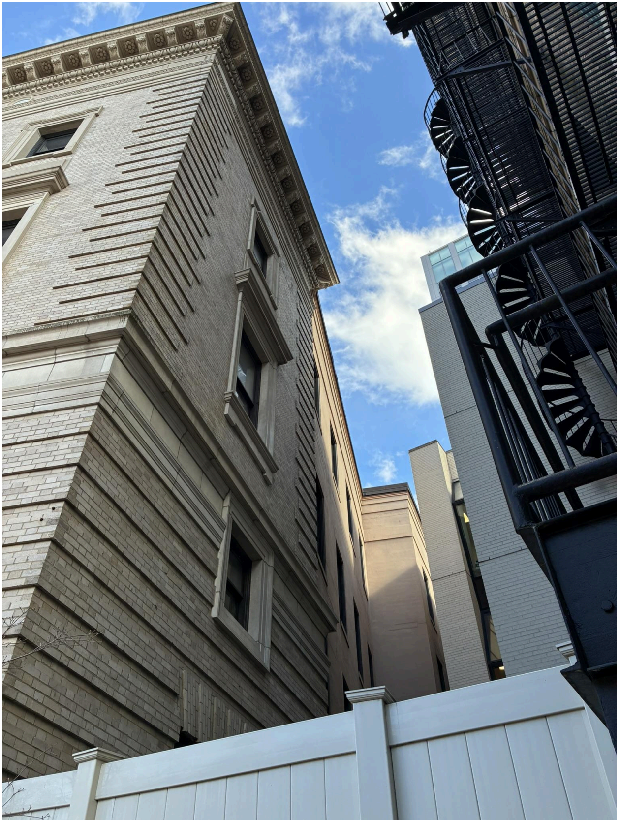
Figure 13. Formal facade treatment wraps around the corner from the Huntington Avenue facade to the southwest (alley) side of the building for one bay. March 2026 by Jennifer Gaugler.
