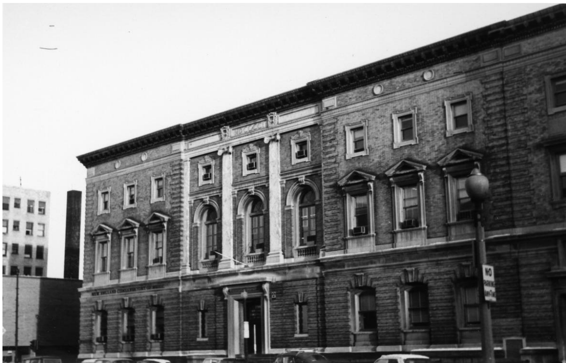
Figure 28. Exterior of New England Conservatory in 1963. 6
