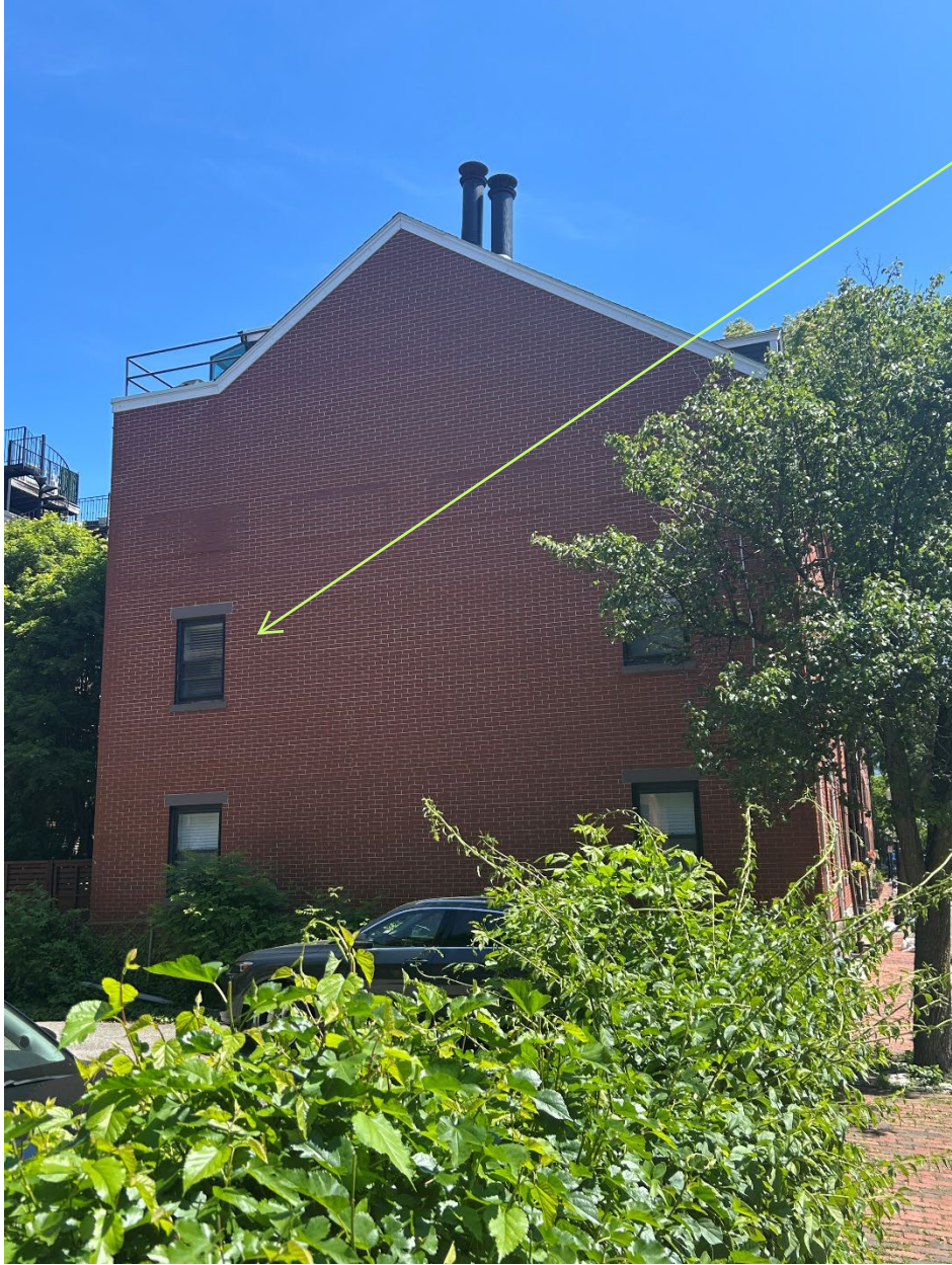
Exterior of 2nd Floor Bedroom window
