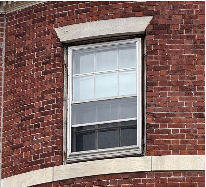
Typical exterior 124 Bay State Road North Elevation window
