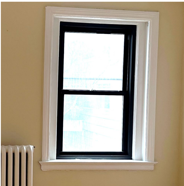
Typical interior 124 Bay State Road South Elevation window
