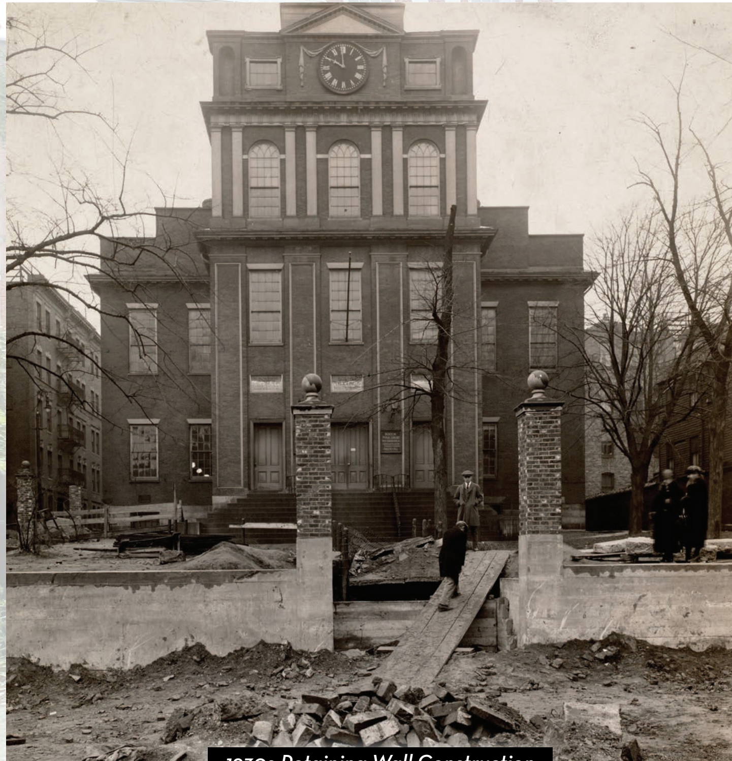
1930s Retaining Wall Construction after Street Lowering
