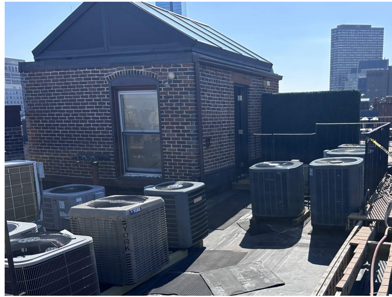
EXISTING COMMON ROOF ENTRANCE
