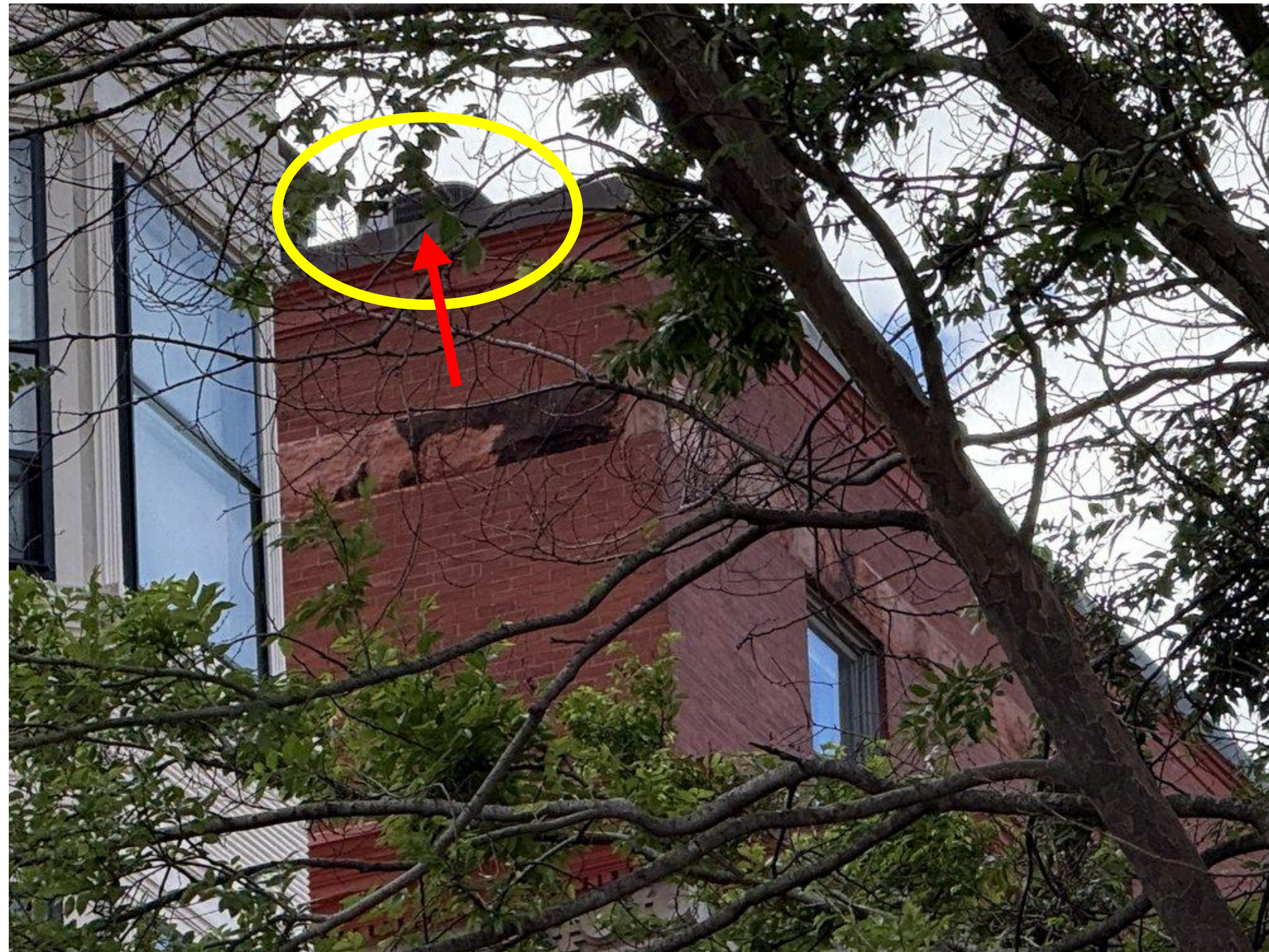
ZOOMED IN VIEW FROM EXETER STREET LOOKING SOUTH - MOCKUP RAILING AND HVAC ARE NOT VISIBLE
