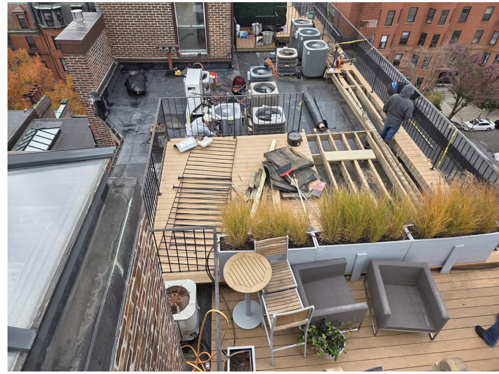
OVERALL VIEW OF EXISTING DECK
