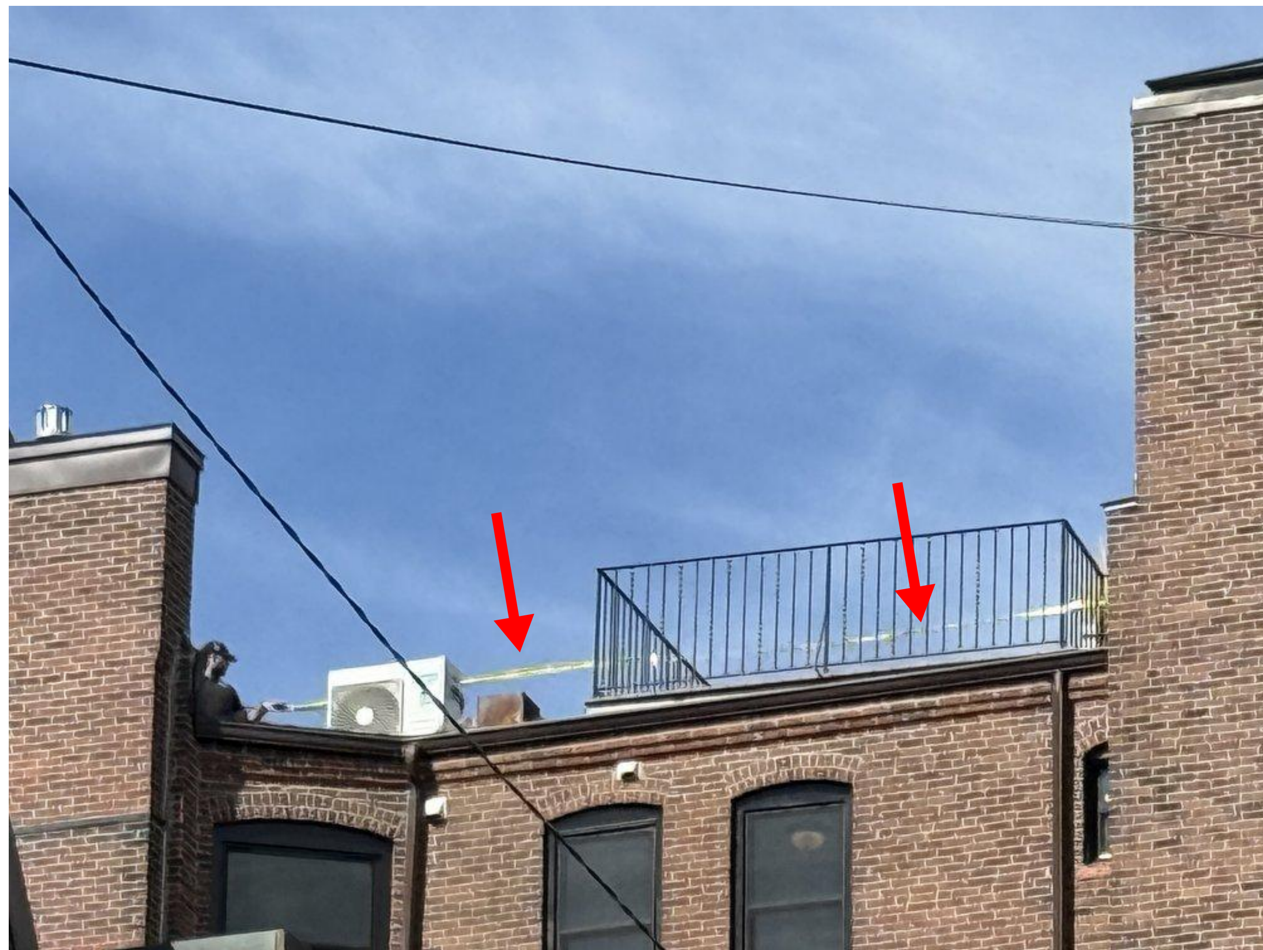
ZOOMED IN VIEW FROM PUBLIC ALLEY LOOKING WEST - MOCKUP RAILING IS PARTIALLY VISIBLE. HVAC CONE IS NOT.
