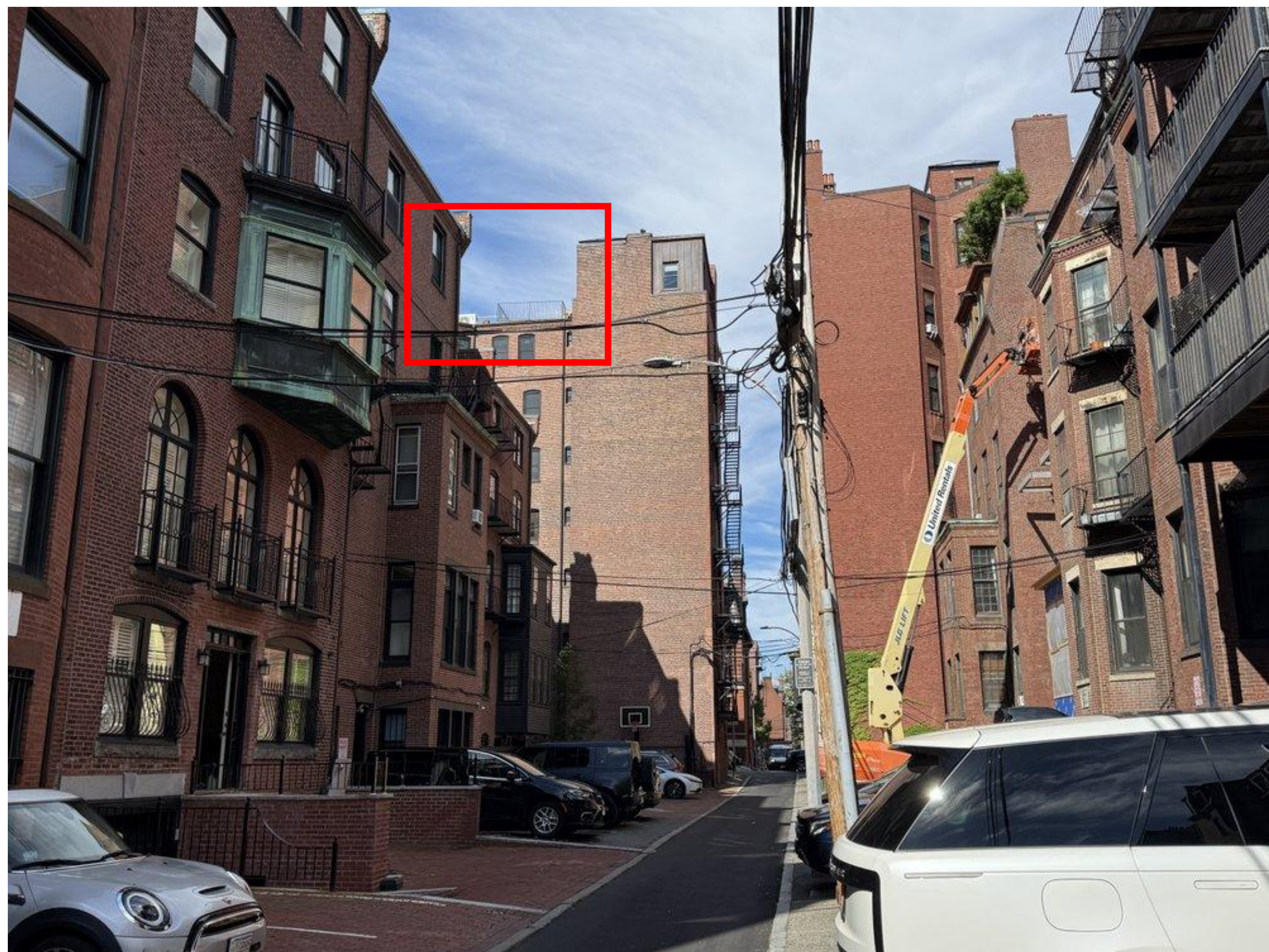
STREET VIEW FROM PUBLIC ALLEY LOOKING WEST - MOCKUP RAILING IS PARTIALLY VISIBLE. HVAC IS NOT.
