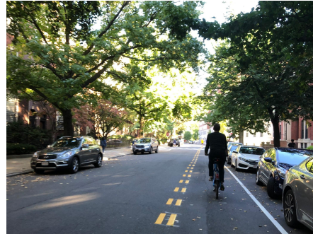
CONTRAFLOW BIKE LANE
