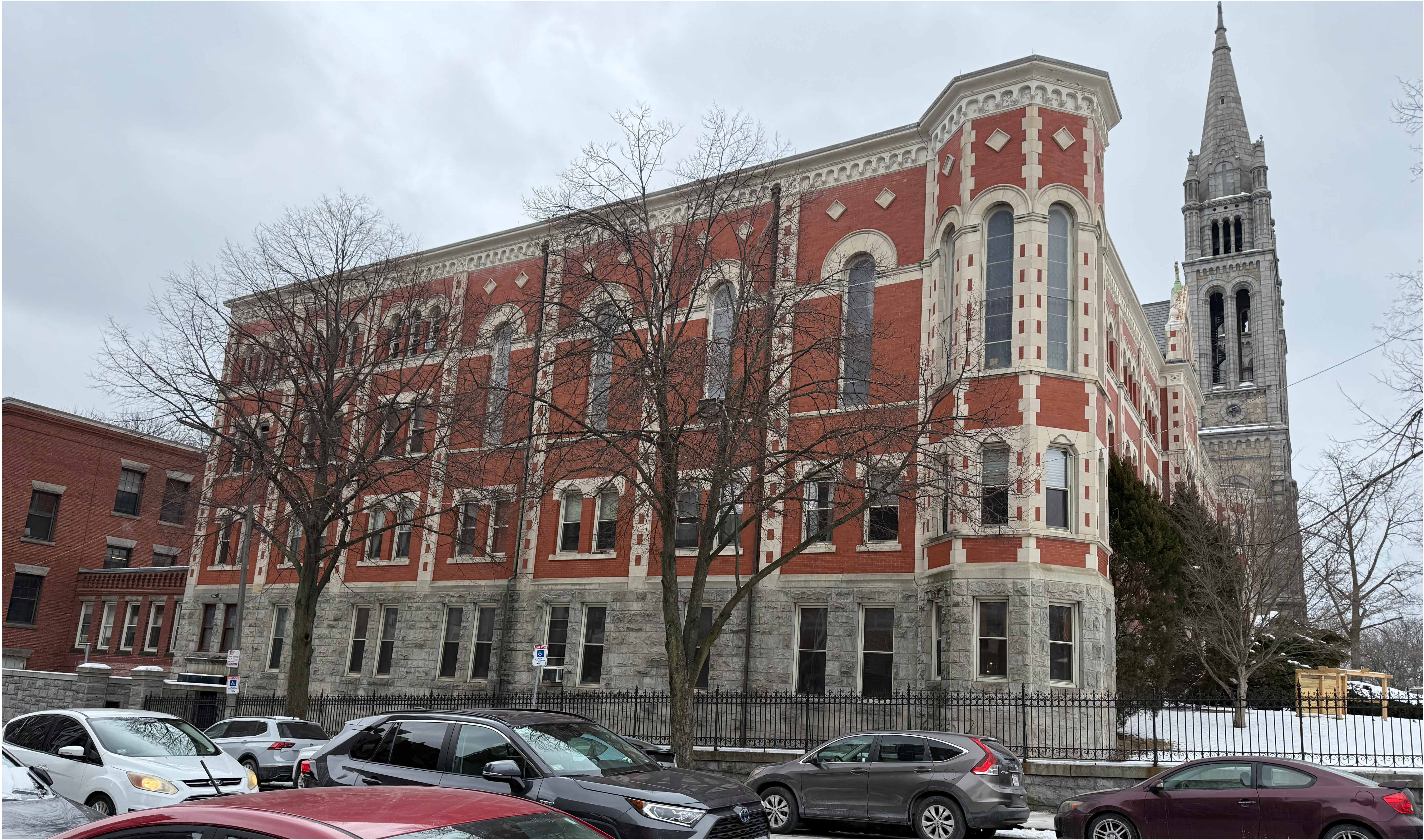
WEST RECTORY FACADE [ST ALPHONSUS ST]
