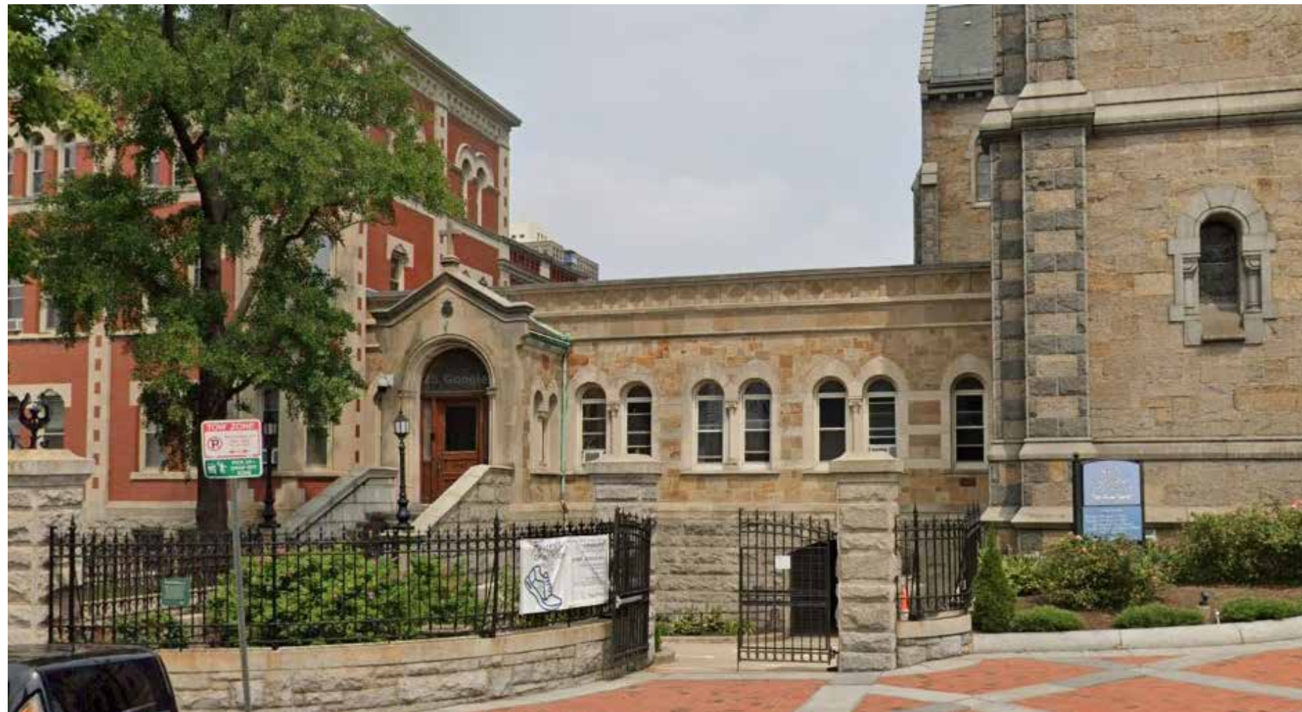
ANNEX Constructed simultaneously with the rectory in 1903
