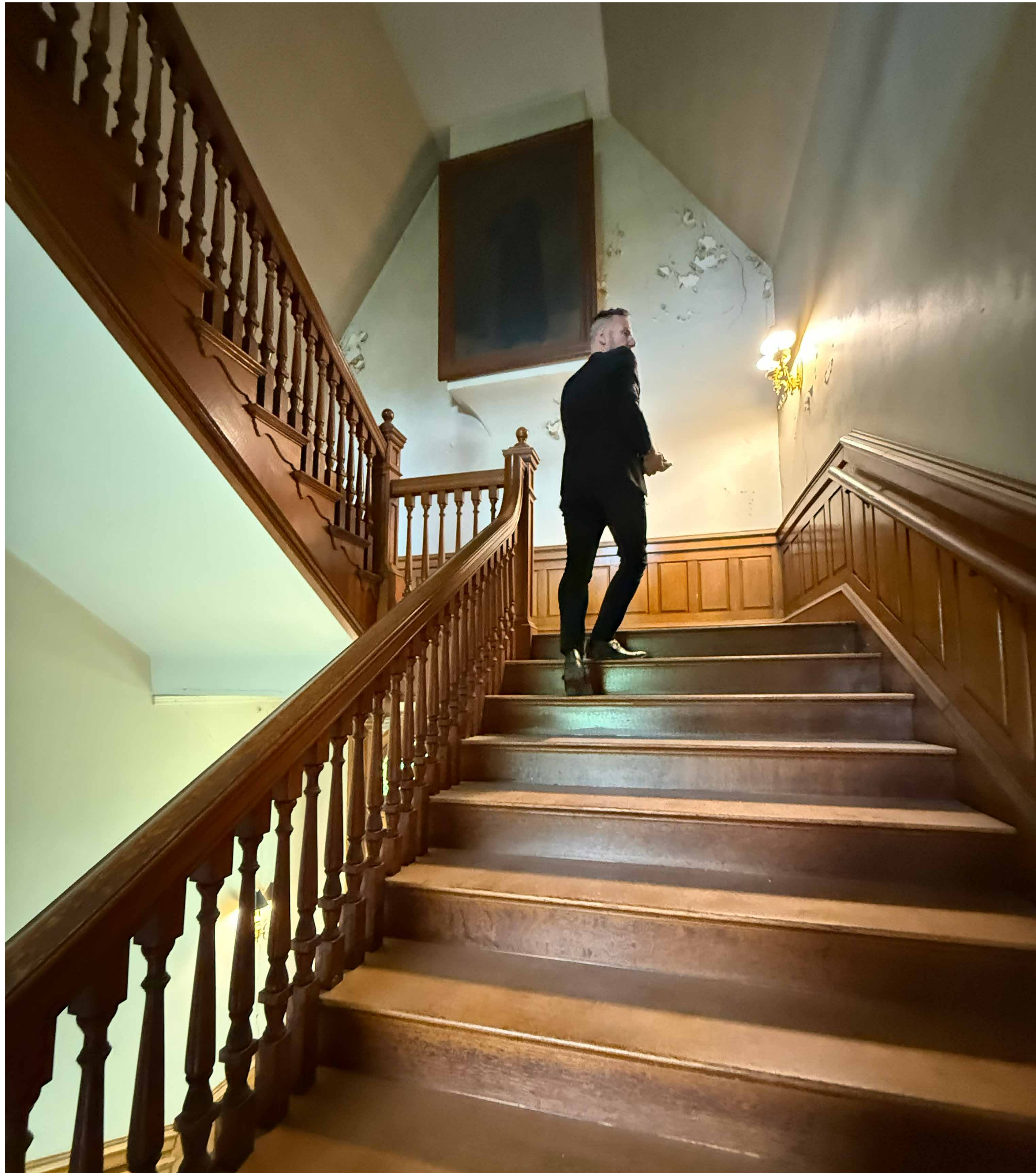
LEVEL 04 & LEVEL 05 PENTHOUSE STAIR CONDITION [INTERIOR VIEW]
