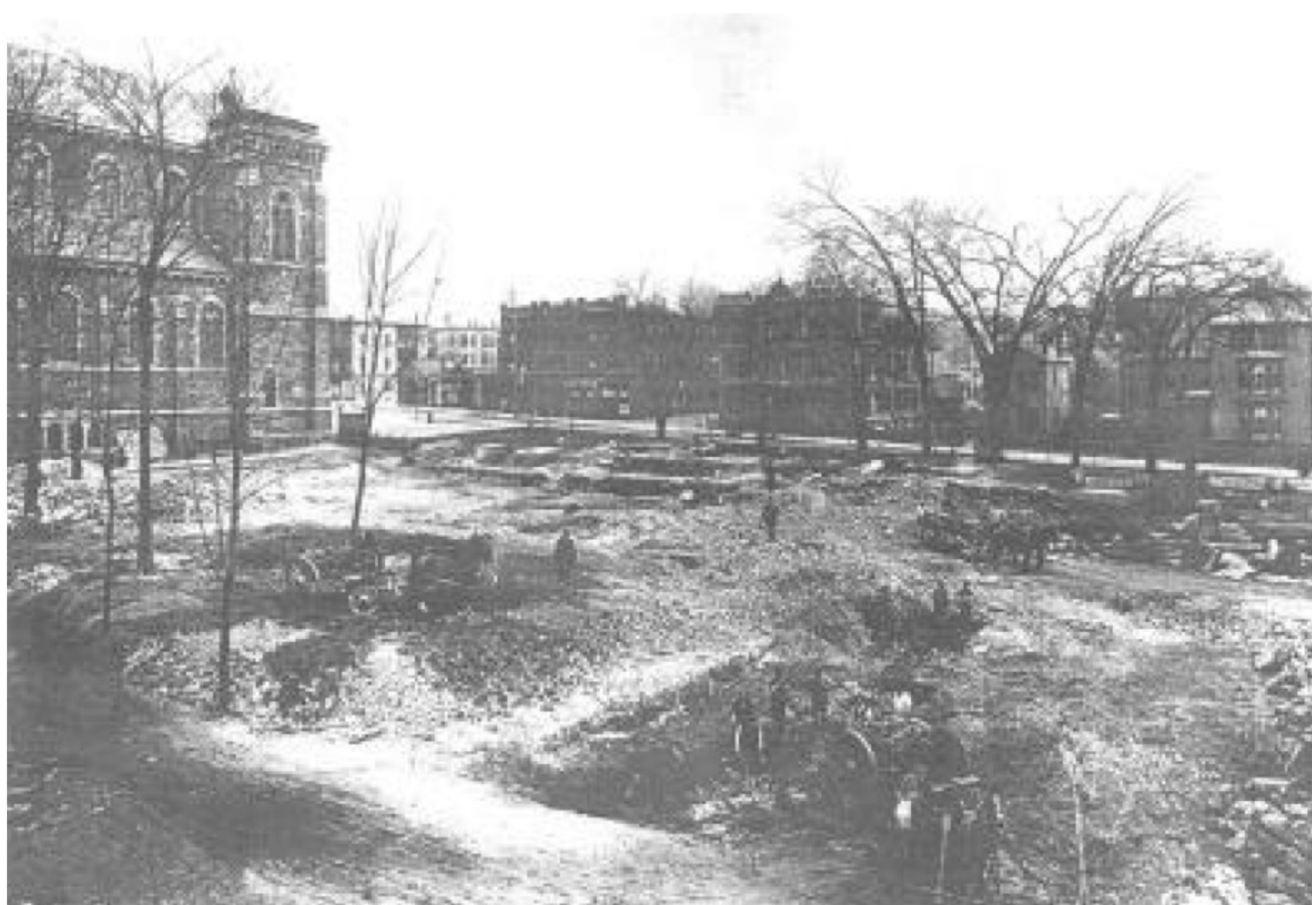
Construction of the Rectory Building
