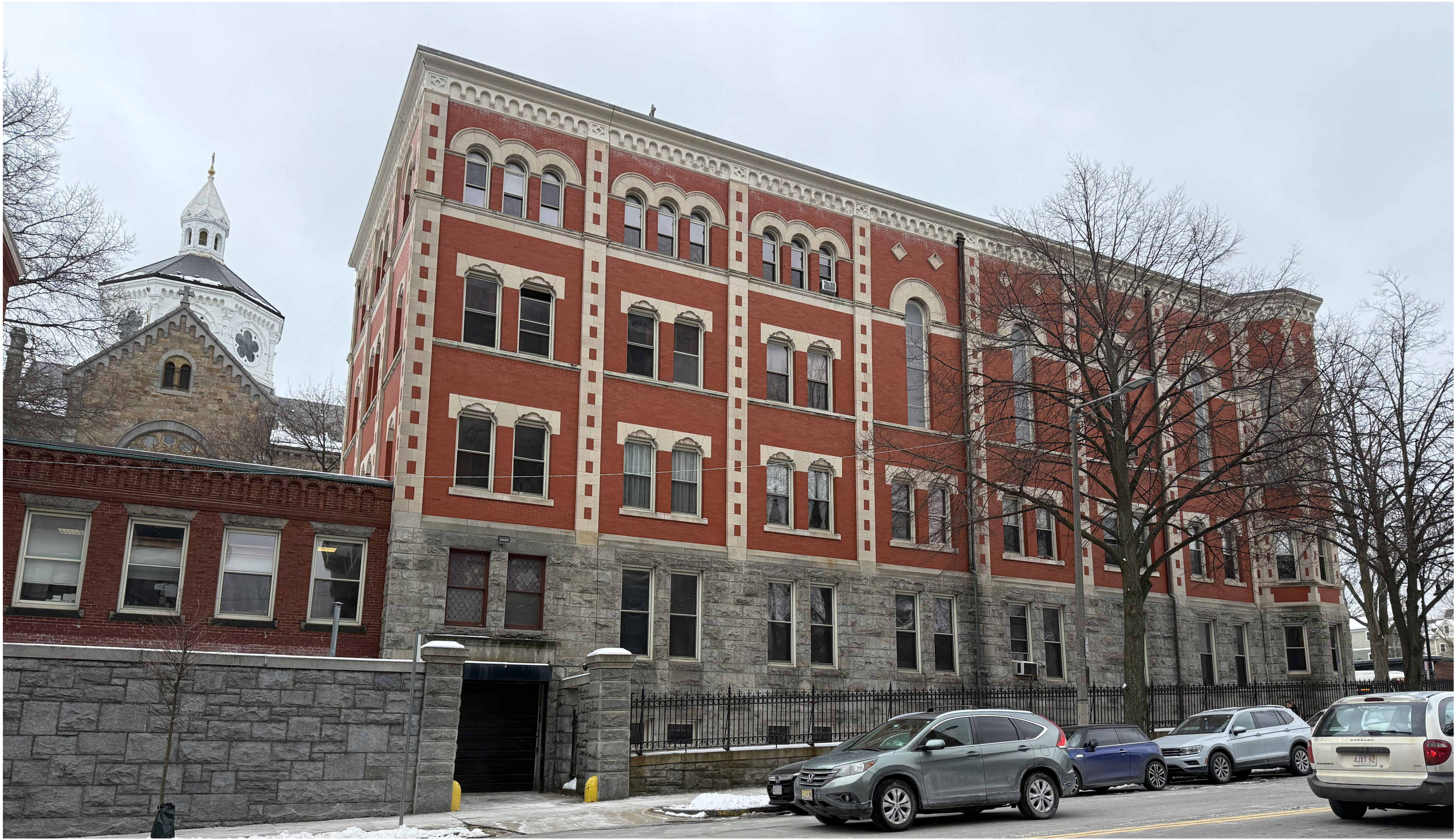
WEST RECTORY FACADE [ST ALPHONSUS ST]
