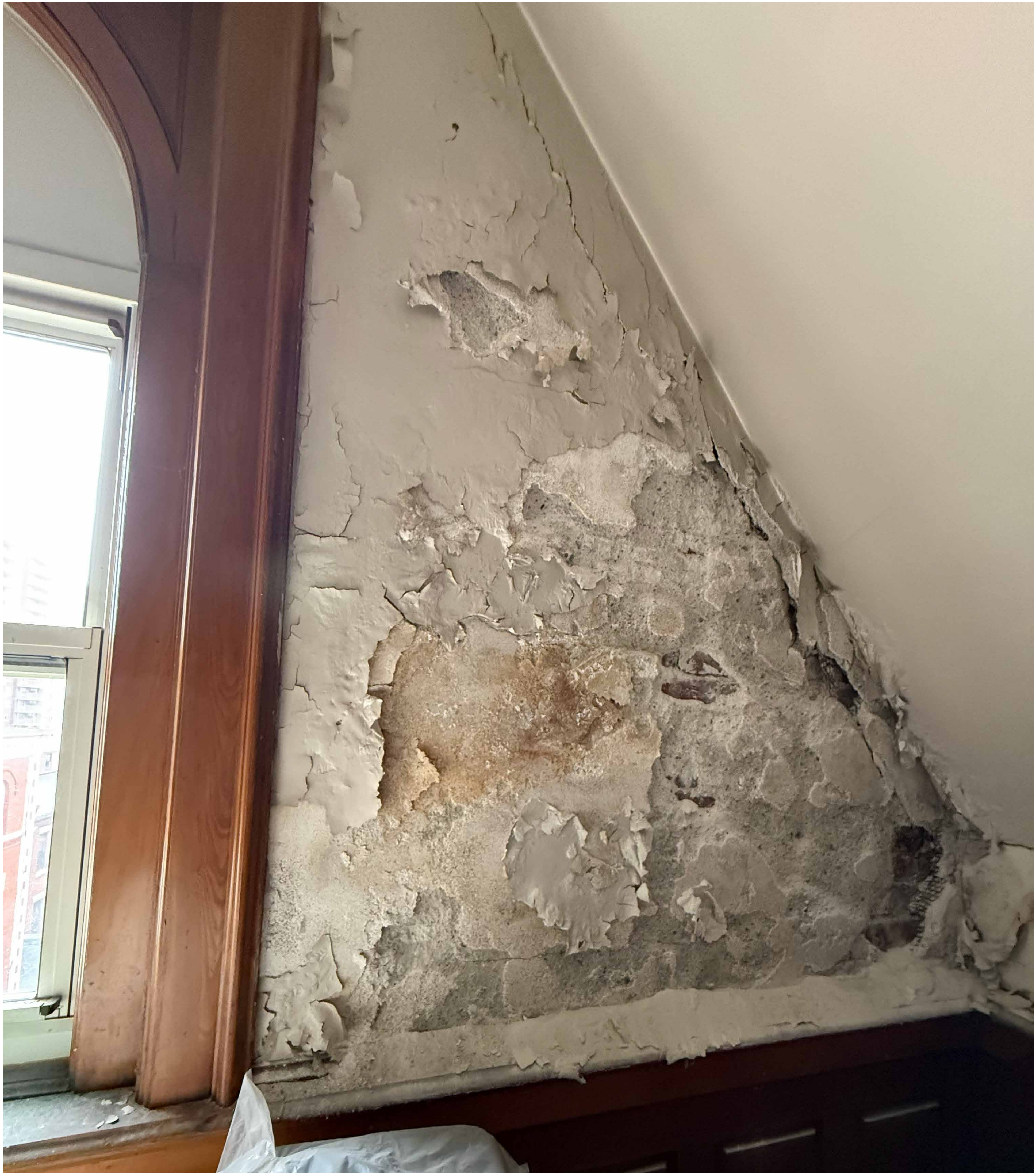
LEVEL 05 PENTHOUSE WALL CONDITION [INTERIOR VIEW]
