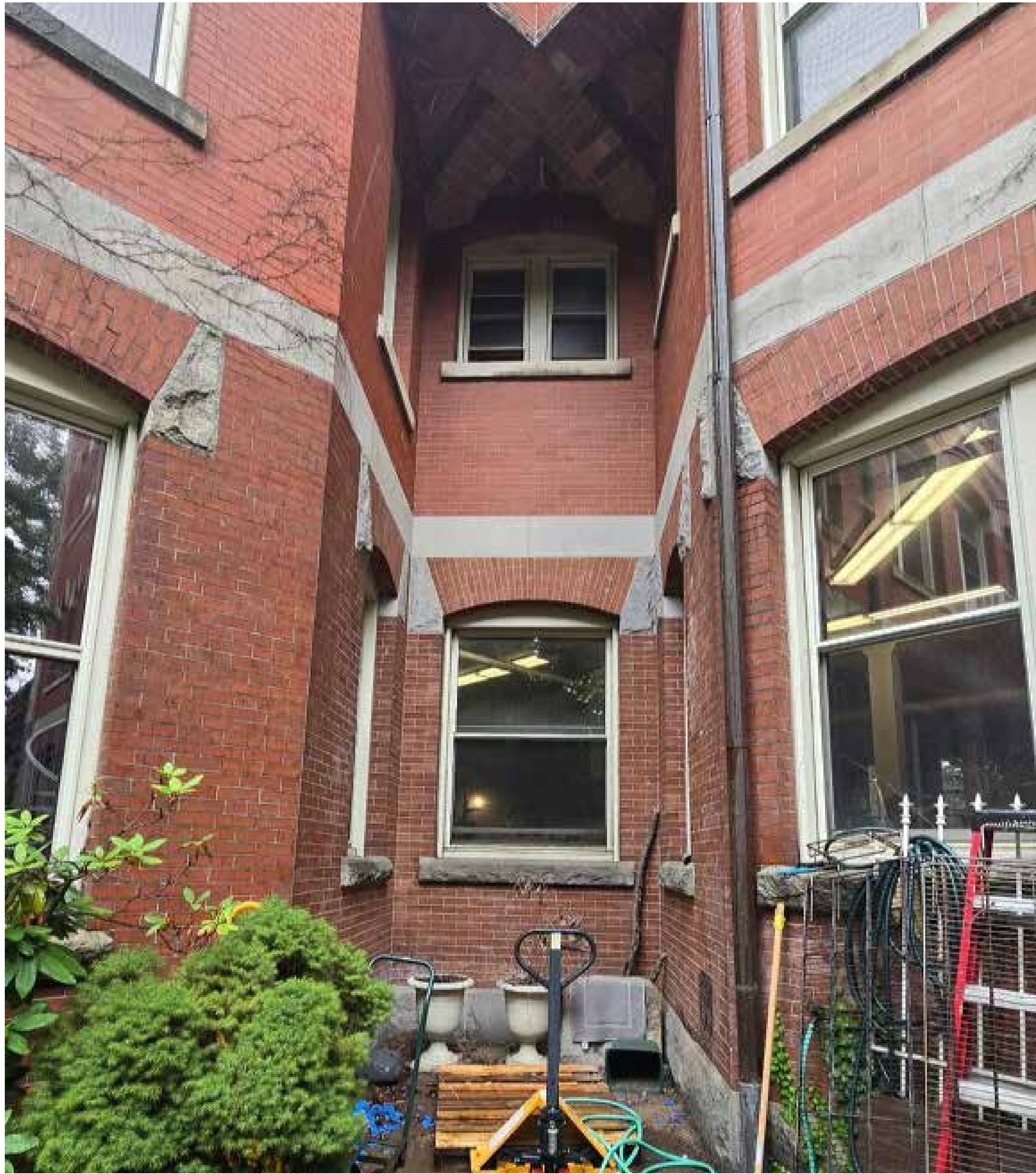
NORTH EAST RECTORY FACADE & INSIDE CORNER CONDITION [COURTYARD VIEW]
