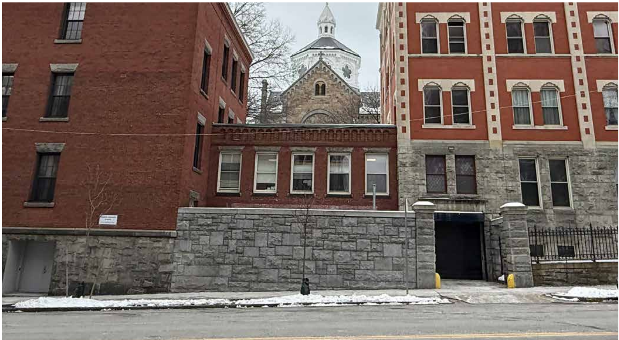
ANNEX Constructed simultaneously with the rectory in 1903
