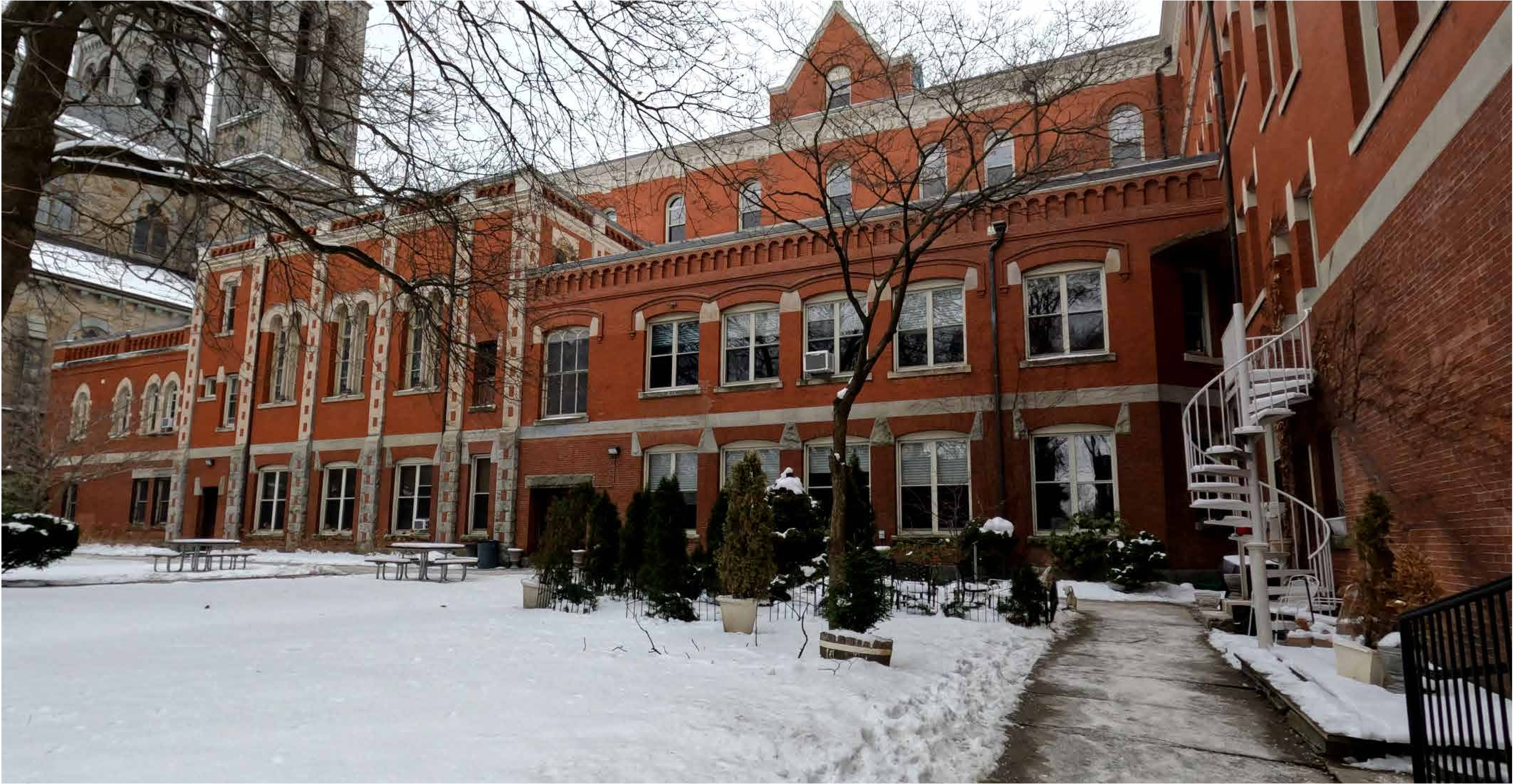
NORTH RECTORY FACADE [COURTYARD VIEW]
