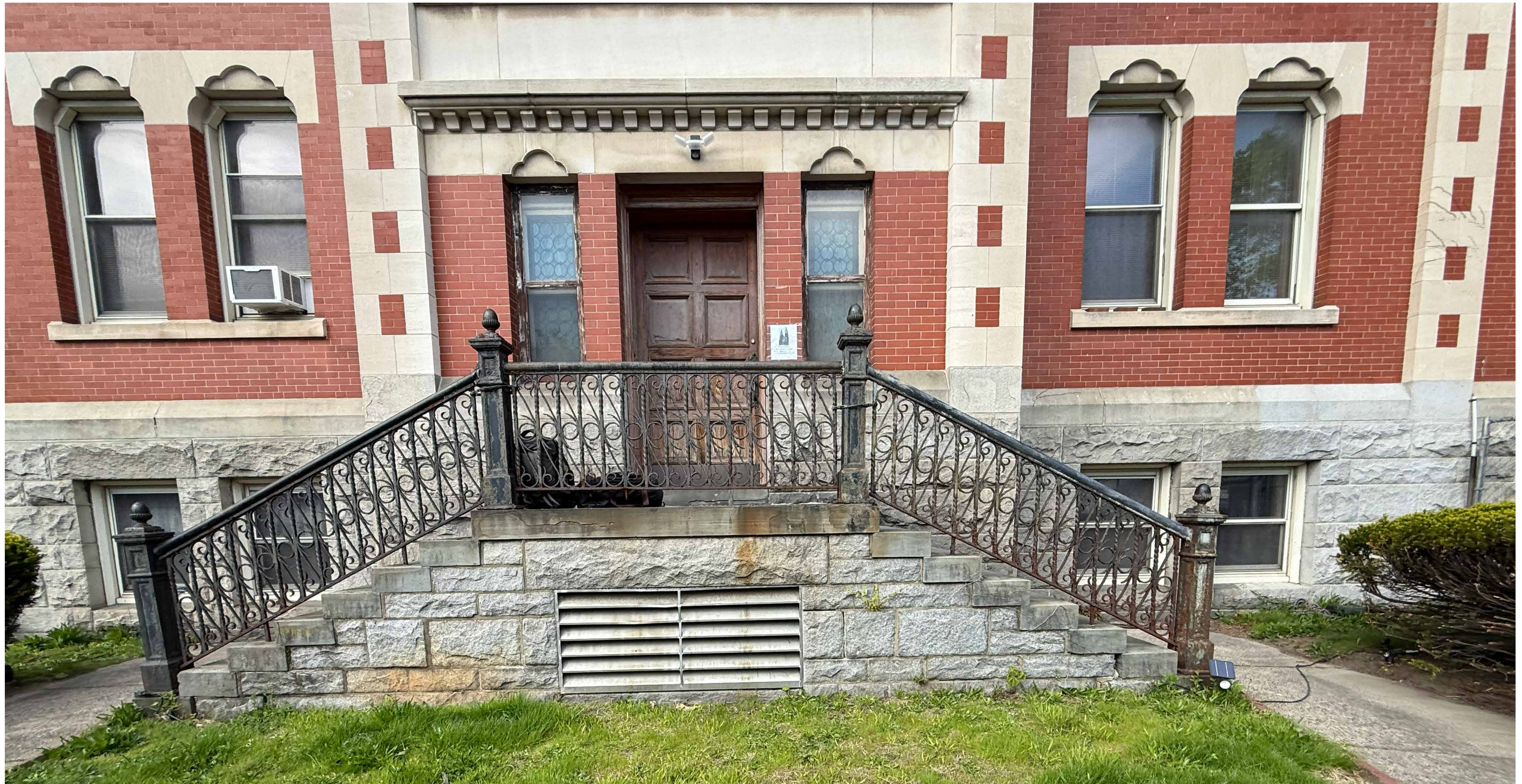
SOUTH RECTORY FACADE [STAIR CONDITION]
