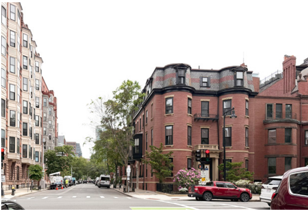
2. VIEW FROM EXETER ST
