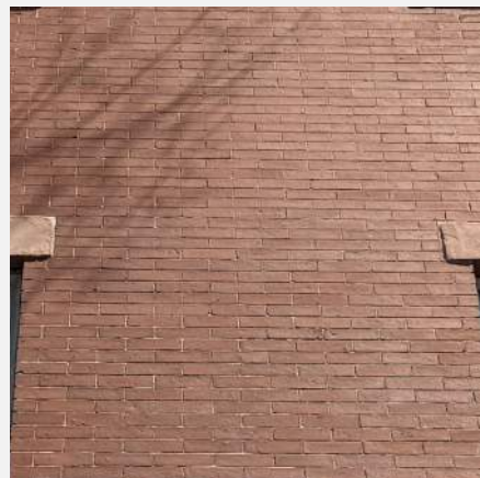
EXISTING BRICK: CLEAN AND REPOINT/REPAIR
