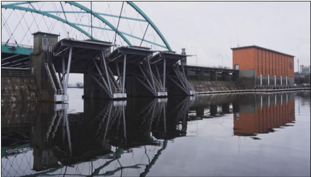
Figure 36. Fox Point hurricane barrier
