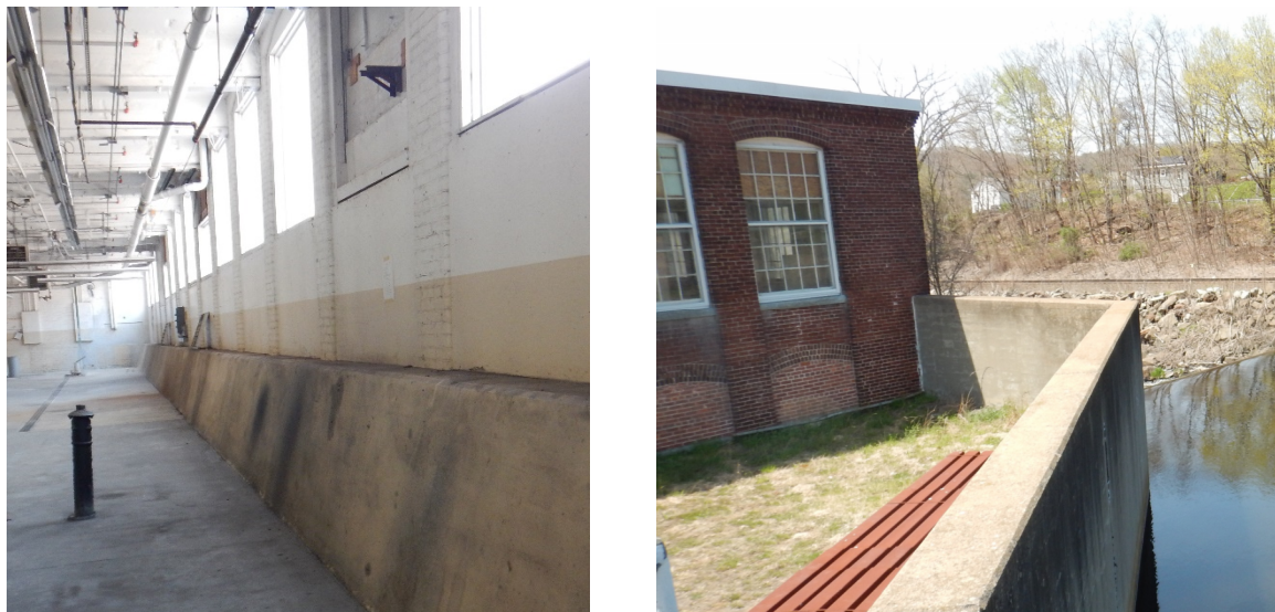
Figure 2: Example of a flood wall integrated with an existing building
