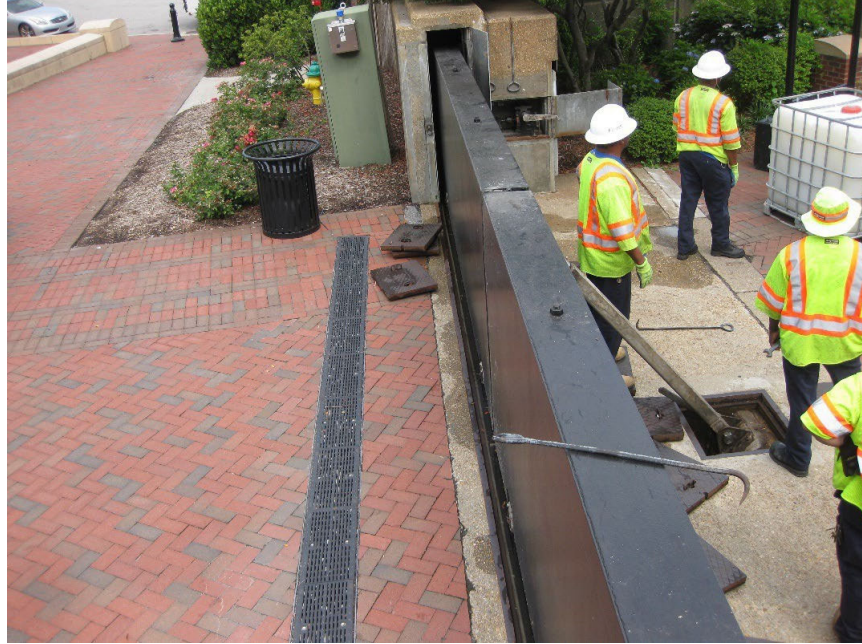
Figure 7: Slide Gate Example (Photo courtesy of USACE Norfolk District)
