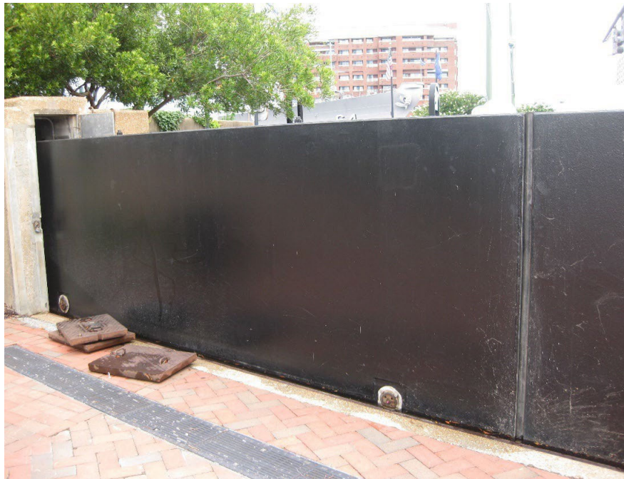
Figure 8: Slide Gate Example (Photo courtesy of USACE Norfolk District)
