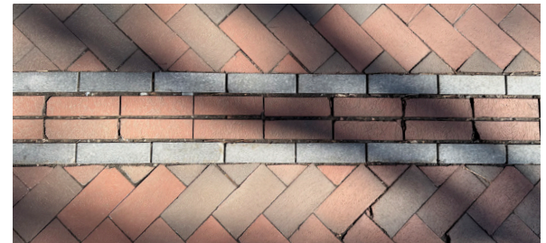
Paul Revere Mall - Paving & Site Elements
