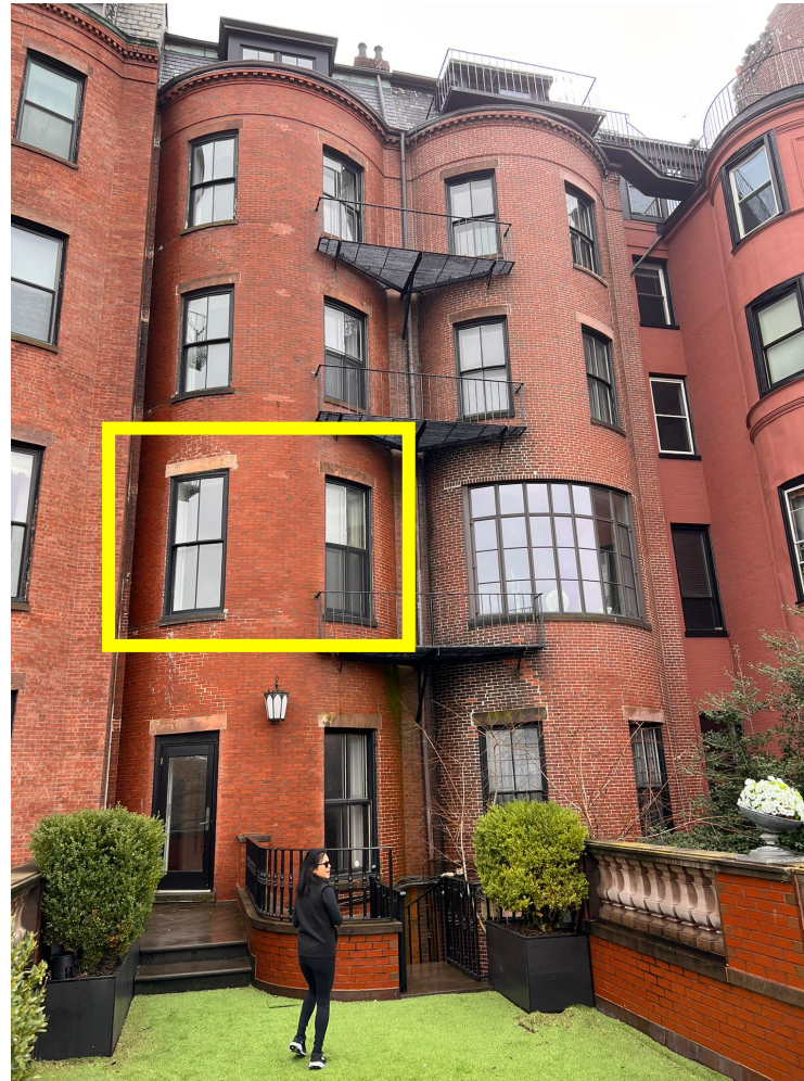
Proposed Work Area, note neighboring steel section window at the sister building at 228 Beacon Street
