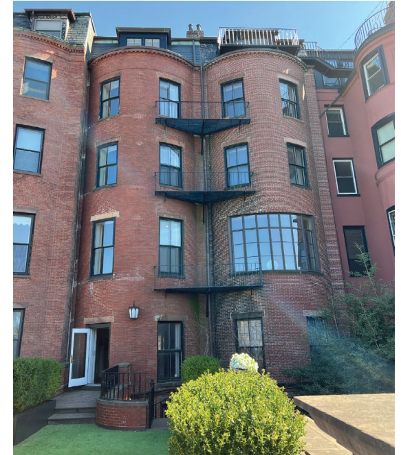
Existing Rear Facade
